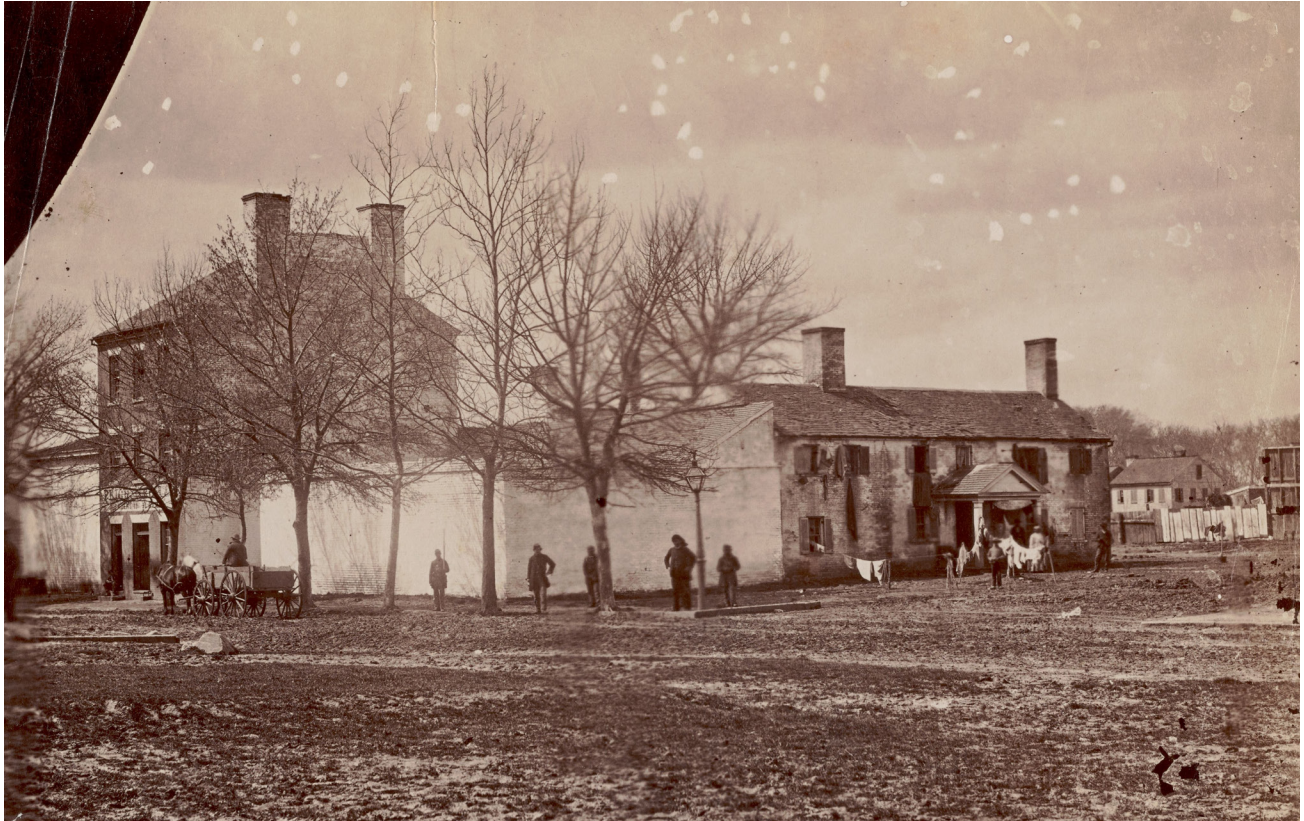
Figure 06: This image of the former slave pen at 1315 Duke Street was taken from the southeast corner of the intersection of Duke and Payne streets. Although it dates to the Civil War period, it is the best historic photograph of the two-story, brick building set back from Payne Street. While this building was likely constructed during Period 2, its original function is not clear. The whitewashed walls of the former women’s yard are clearly visible in this image, as is the shed roof that partially covers the space. [Slave pen, Alexandria, VA, Matthew Brady, 1861-1865, Prints and Photographs Division, Library of Congress]
