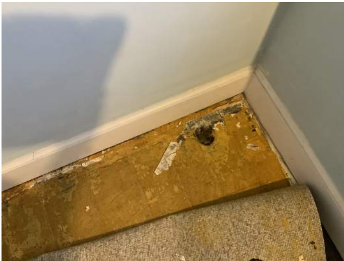
Figure PR4-1: Detail of historic wood flooring located under existing carpet .
