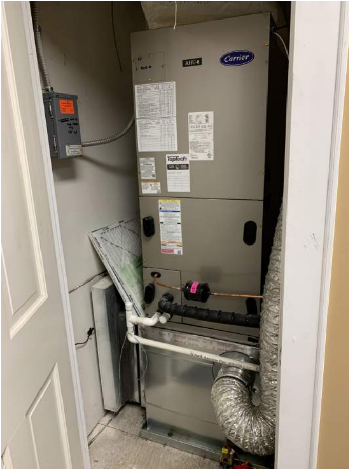
Mechanical Closet 210A
