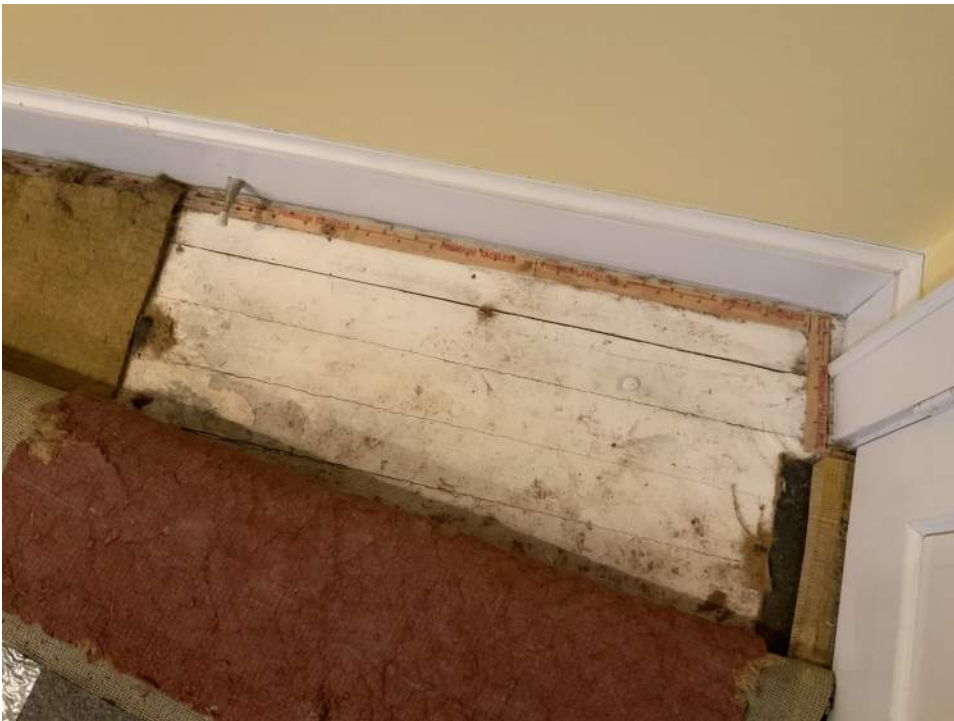
Figure PR13-1: Detail of historic wood flooring located under existing carpet .
