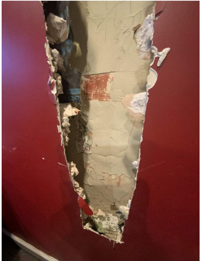
Figure PR12-2: Detail of historic plaster finishes found at investigative probe #12.
