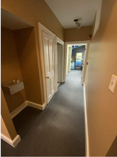
Corridor 305A, looking east
