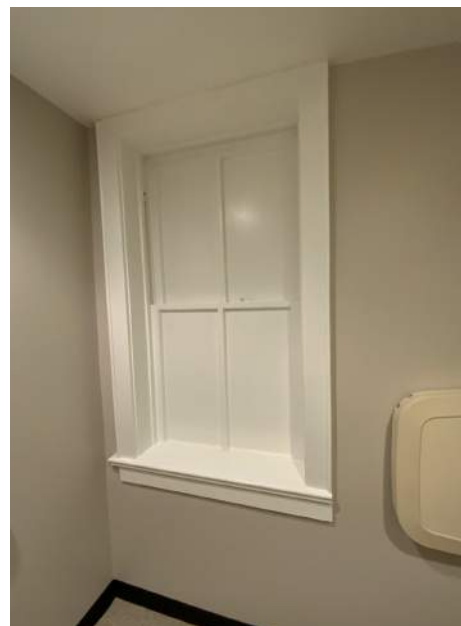
Restroom 108, East Elevation
