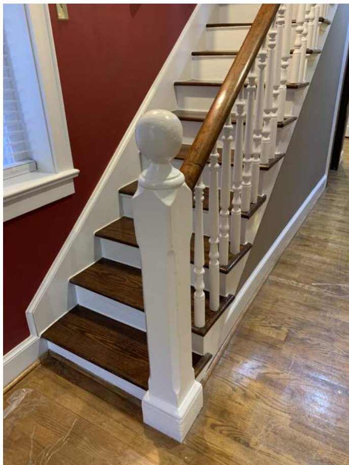
Stair 1, First Floor
