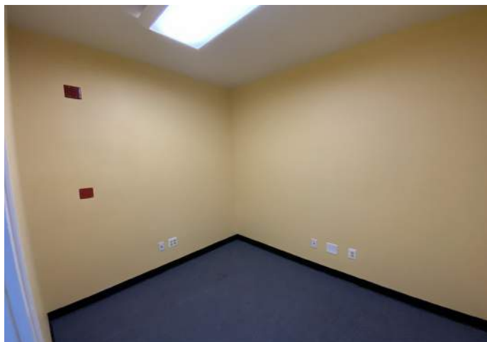
Office 113, North and East Elevations
