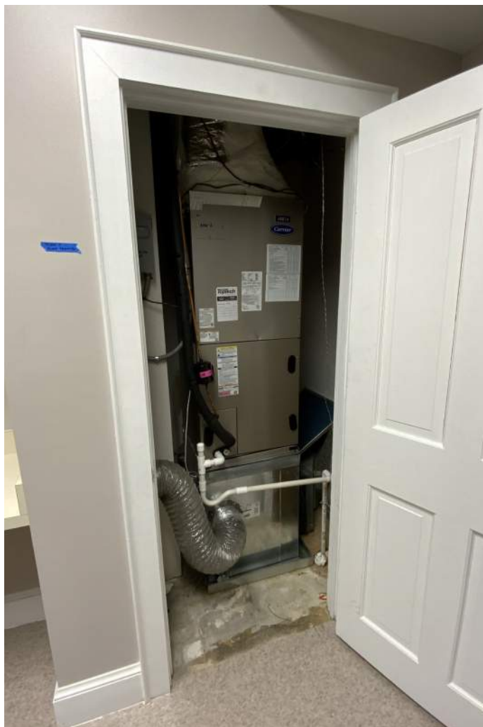
Mechanical Closet 110A
