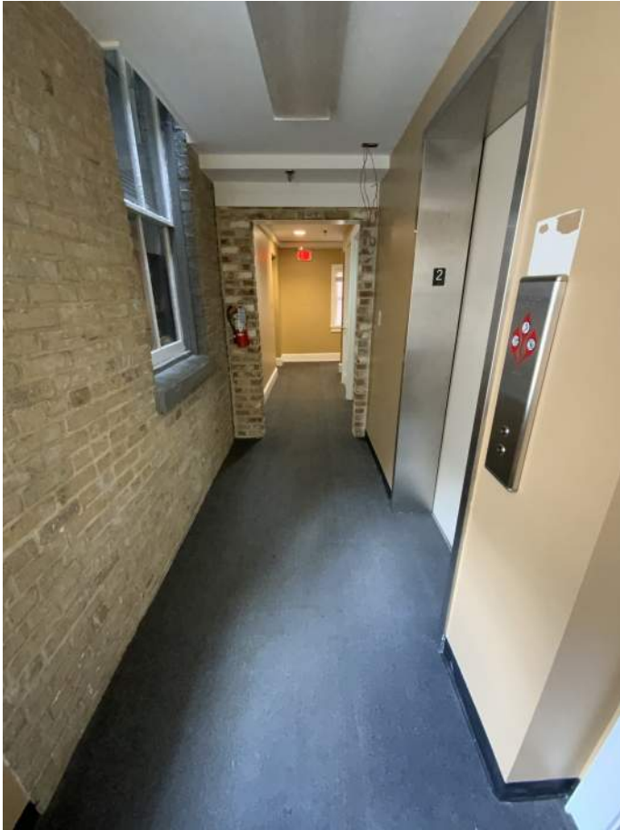
Corridor 205B, West Elevation
