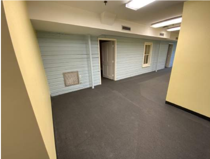
Open Workspace 309, West Elevation
