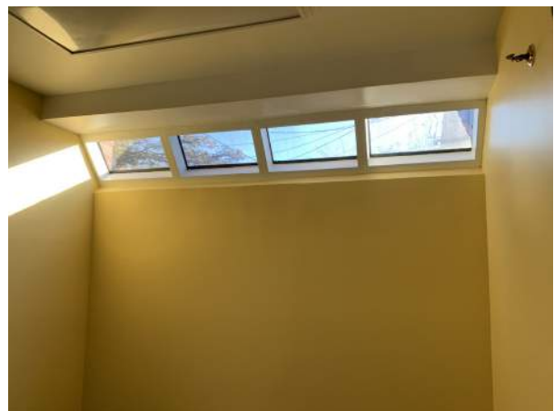
Figure 2C-8: Sloped skylight at first and second floor of 1985 Addition.
