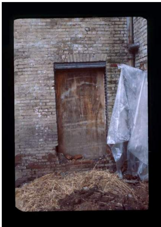
Figure 34: Image of Window 105 c.1980.
