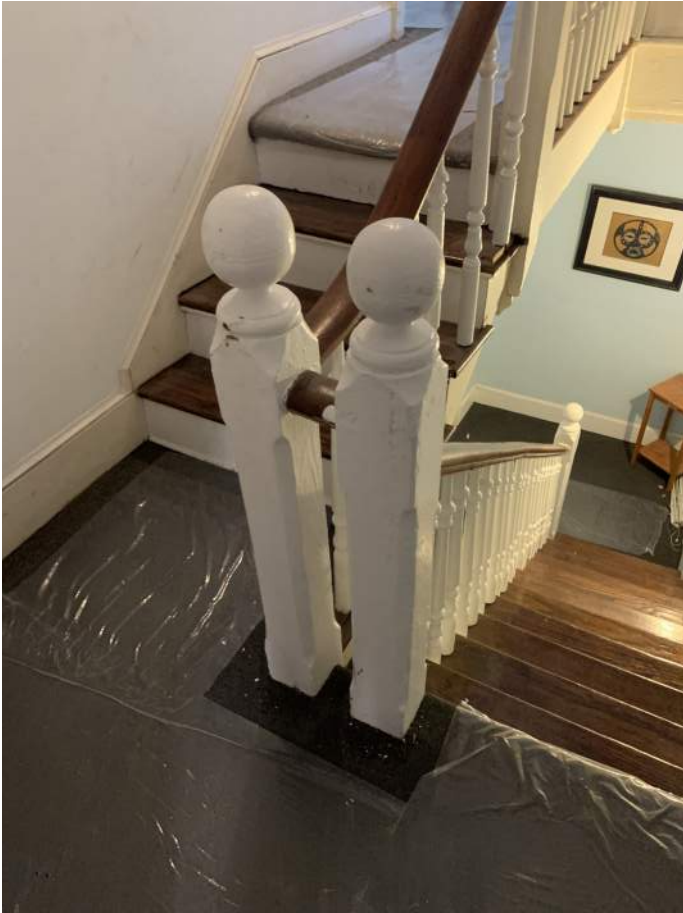
Stair 1, Intermediate Landing between Second and Third Floors
