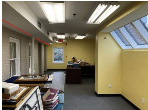
Figure 2C-7: Second Floor interior, 1980s addition, looking north. Interior beam line highlighted in red.
