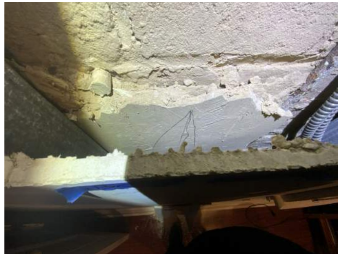
Figure PR7-2: Detail of historic plaster finishes found at investigative probe #7.
