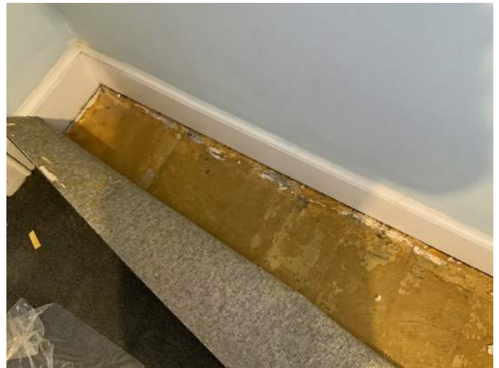
Figure PR4-2: Detail of historic wood flooring located under existing carpet .
