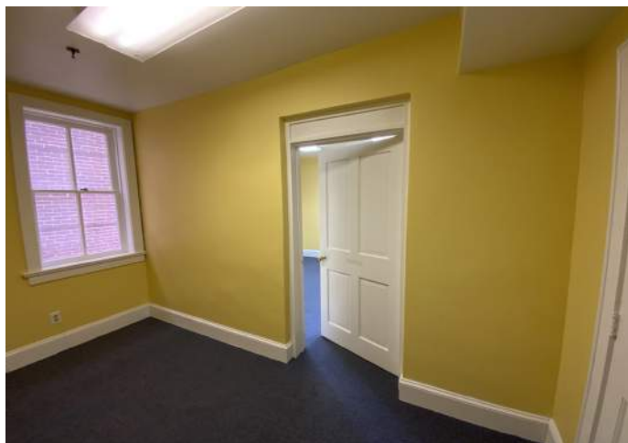
Office 114, North Elevation
