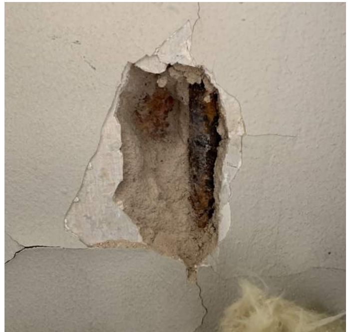
Figure PR10-2: Detail of historic plaster finishes found at investigative probe #10.
