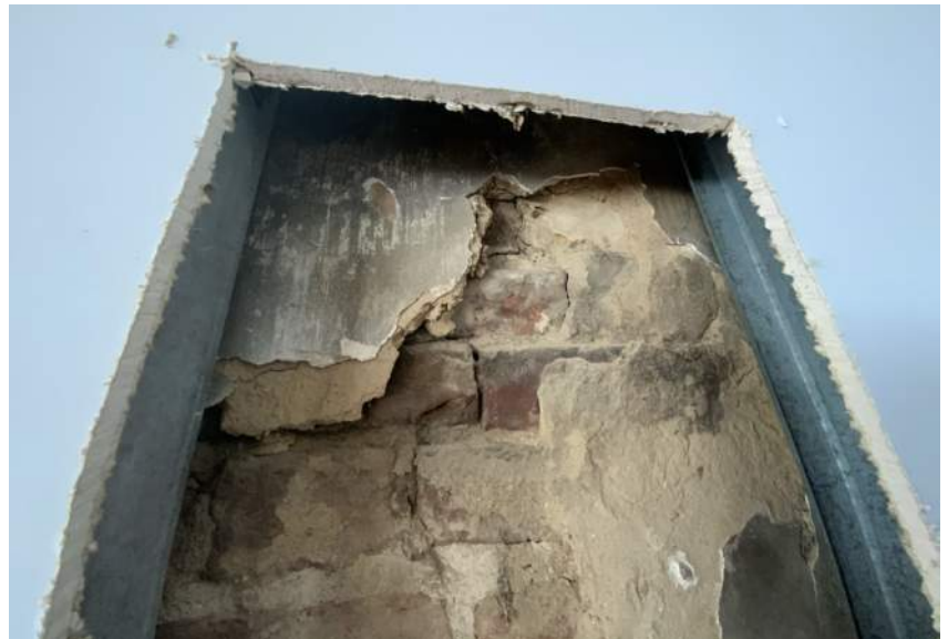
Figure PR6-2: Detail of historic plaster finishes found at investigative probe #6.
