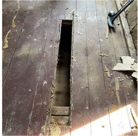
Figure 2D-16: Probe into wood floor at fourth floor/mezzanine.
