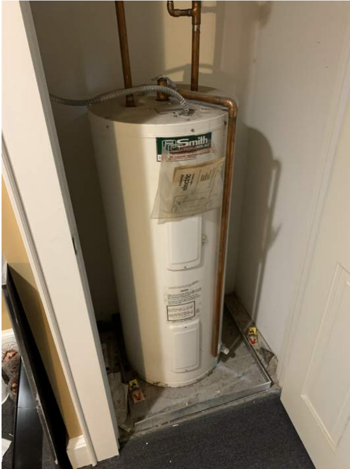
Hot Water Heater Closet 207
