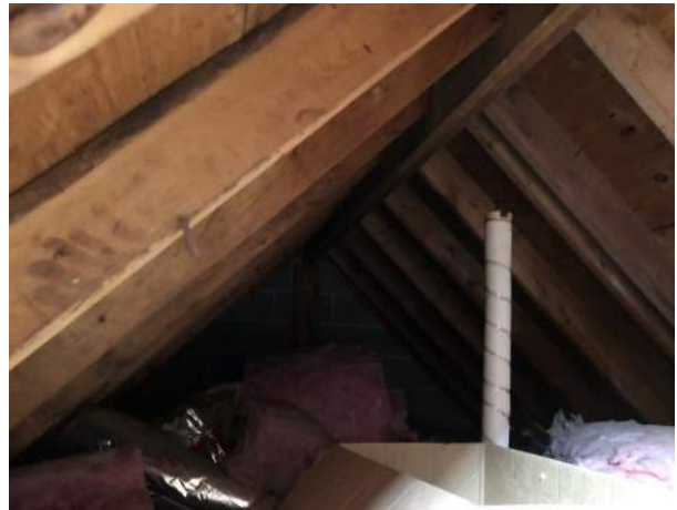
Figure 2C-11: Gabled portion of roof at northeast corner of 1985 Addition.
