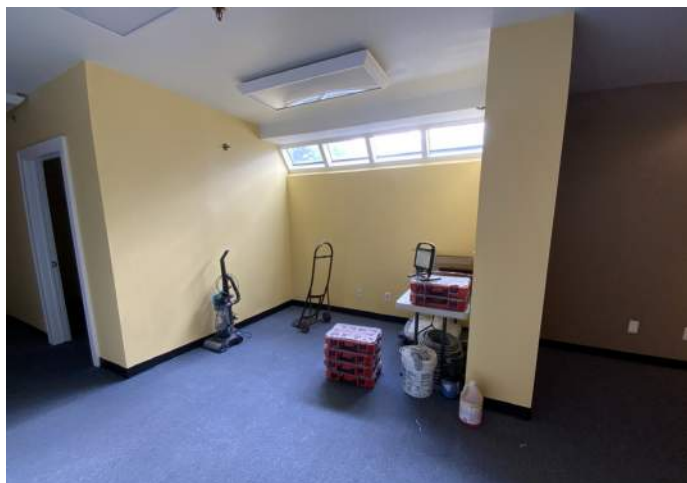
Open Workspace 111, East Elevation
