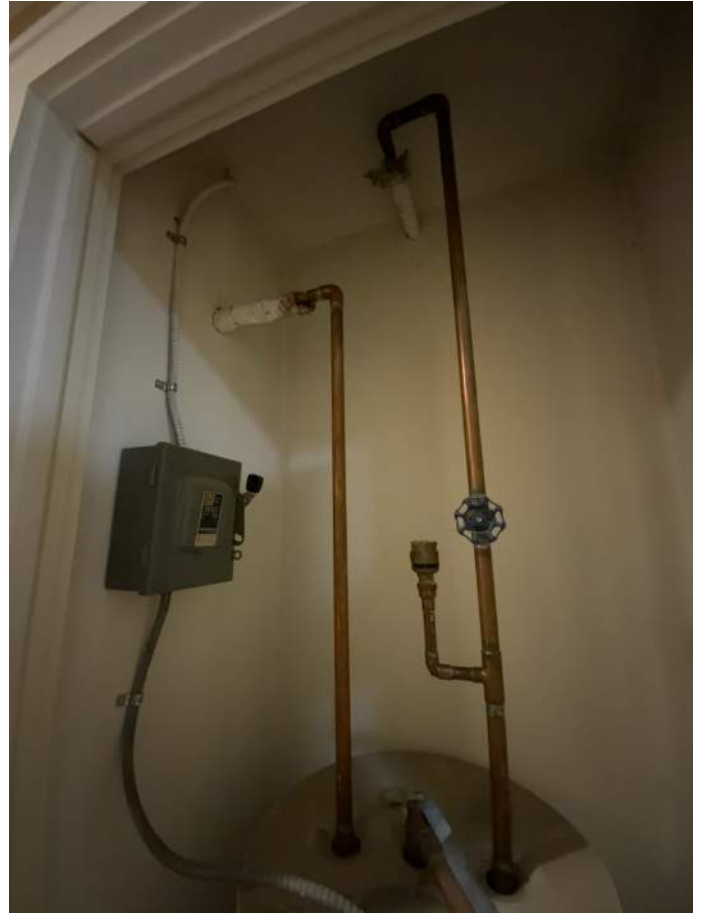
Hot Water Heater Closet 207
