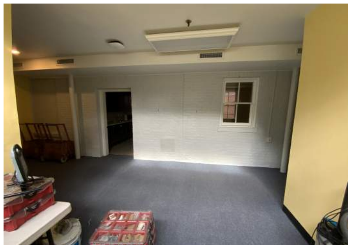
Open Workspace 111, West Elevation
