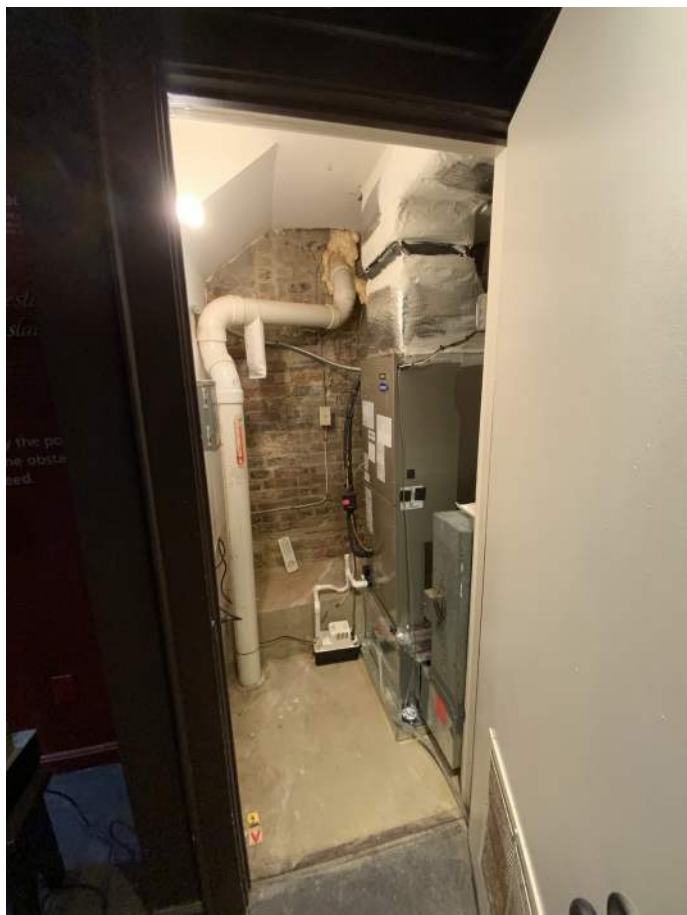
Mechanical Closet 002A
