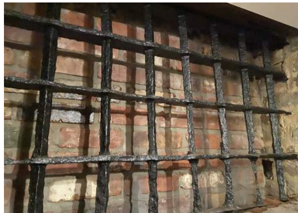
Figure 2C-14: Wrought iron grating within basement
