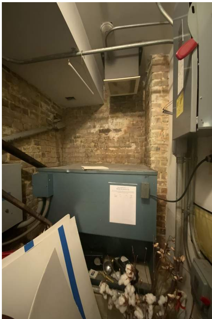
Elevator Machine Room 002B
