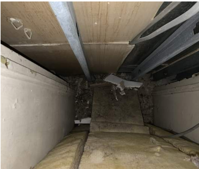
Figure PR15-1: Prior door opening located within in the north wall of the South Block.
