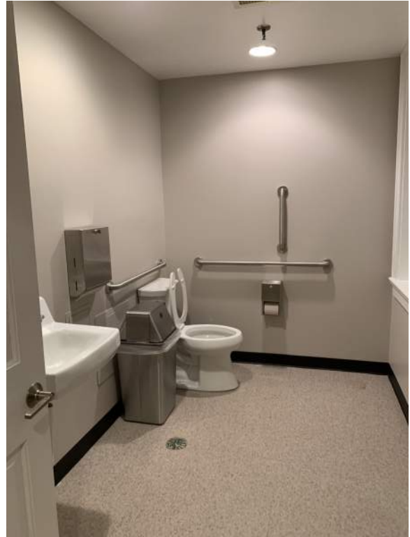
Figure 2D-4: Recently renovated restroom at first floor provides accessible accommodations.
