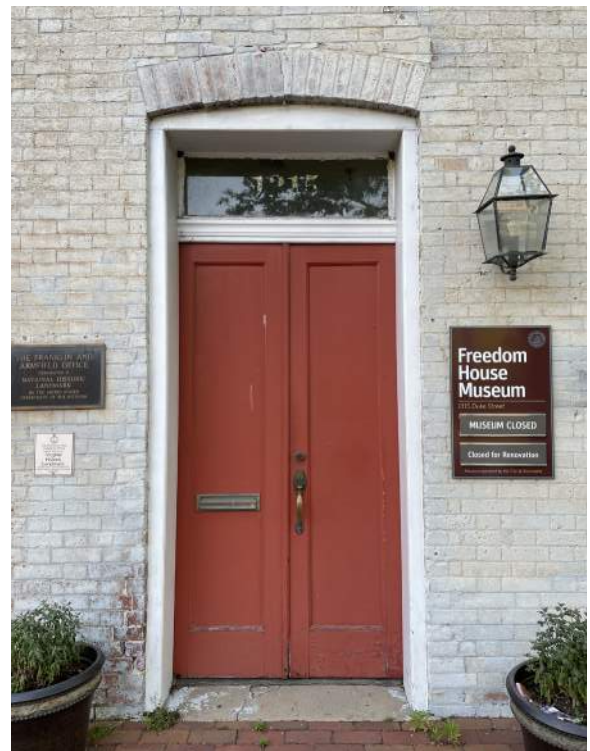
Figure 2D-3: Primary historic entry does not comply with accessibility standards and required modifications to provide equal access.
