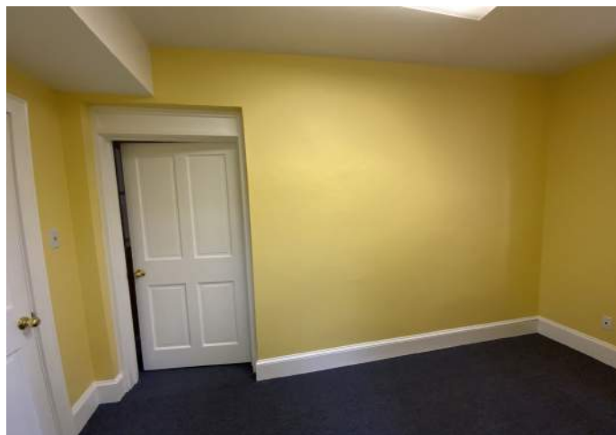
Office 114, South Elevation
