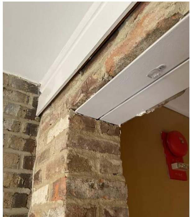
Figure 2C-12: New masonry opening with steel angle lintel.
