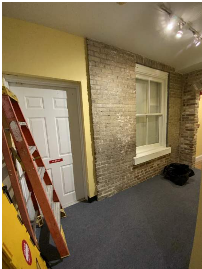
Corridor 105B, South Elevation
