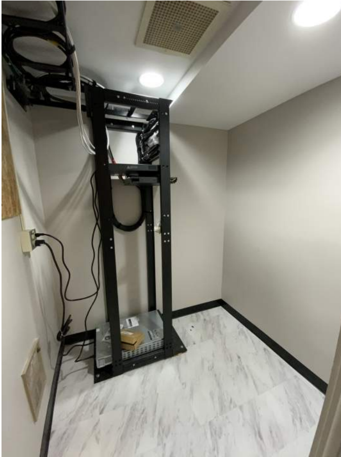
Server Room 206, North Elevation
