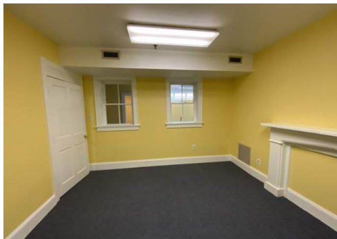
Office 112, East Elevation
