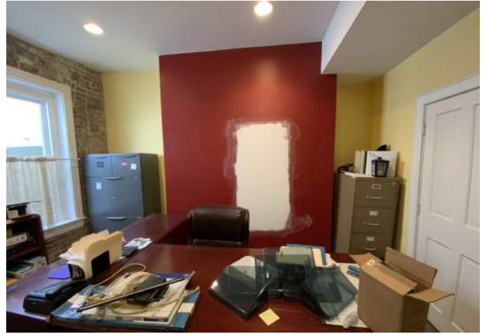
Office 304, East Elevation
