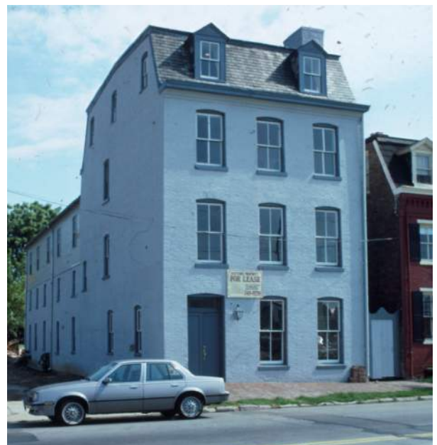
Figure 2B-21: View of 1315 Duke Street after the renovation in 1985. [Office of Historic Alexandria]
