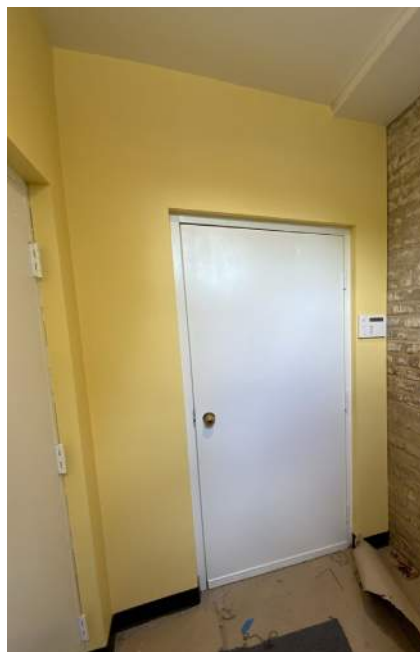
Vestibule 117, South Elevation
