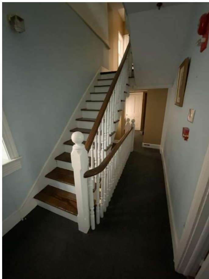
Stair 1, Second Floor Landing
