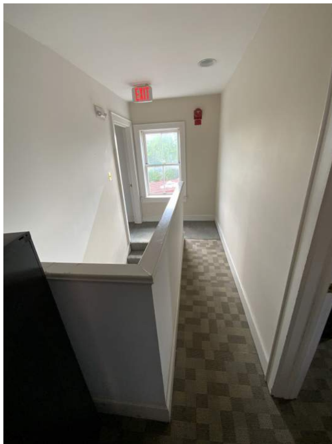
Corridor 402, View looking east with Stair 2 on the left.
