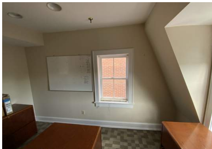
Office 404, West Elevation
