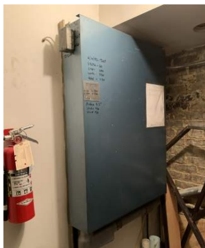
Elevator Machine Room 002B
