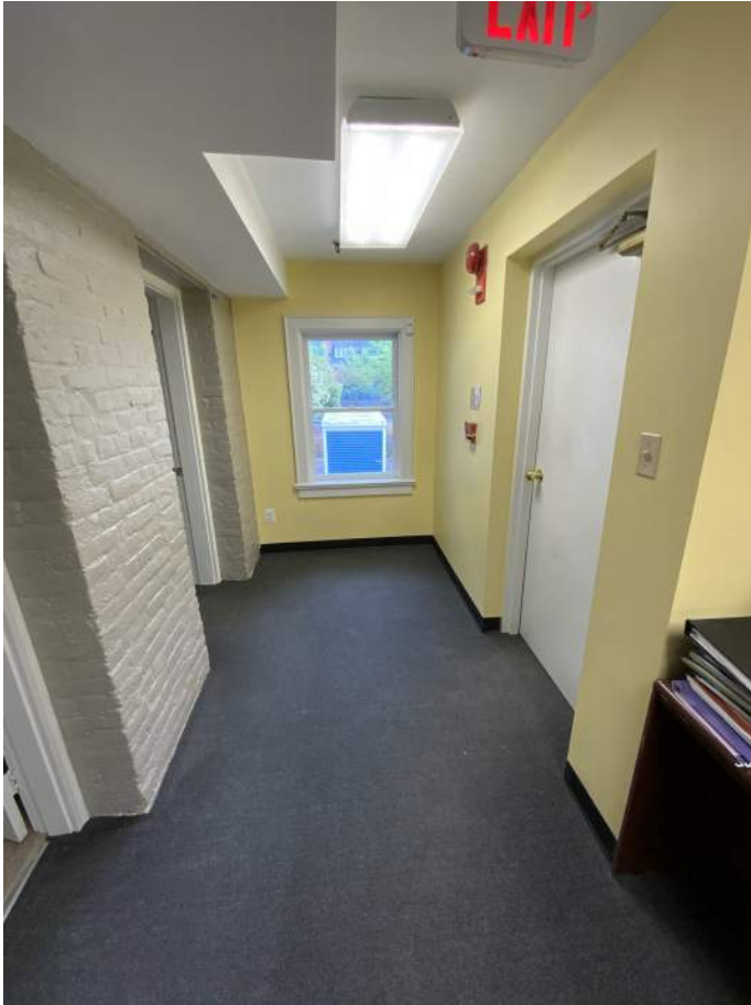
Vestibule 217, North Elevation
