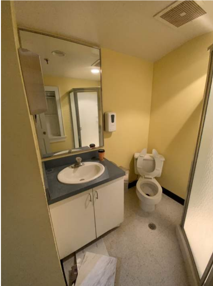
Restroom 208, West Elevation
