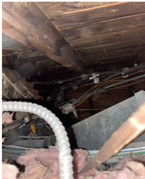
Figure 2C-9: Northwest portion roof, viewed above ceiling light.
