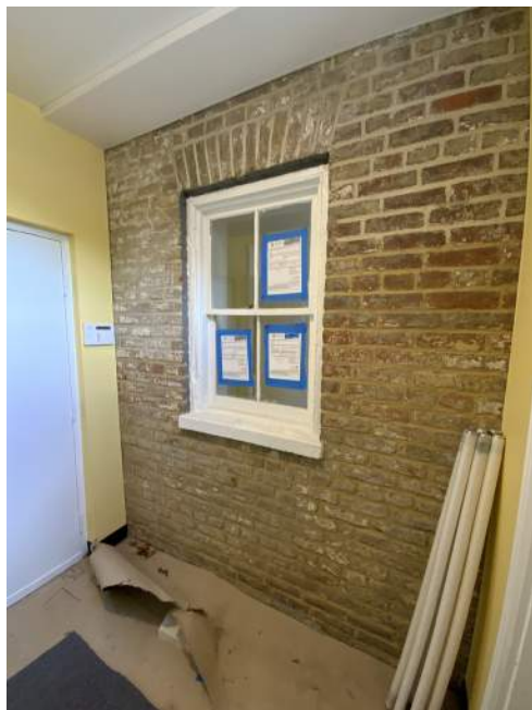
Vestibule 117, West Elevation
