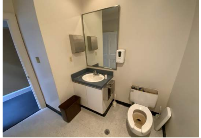
Restroom 308, West Elevation
