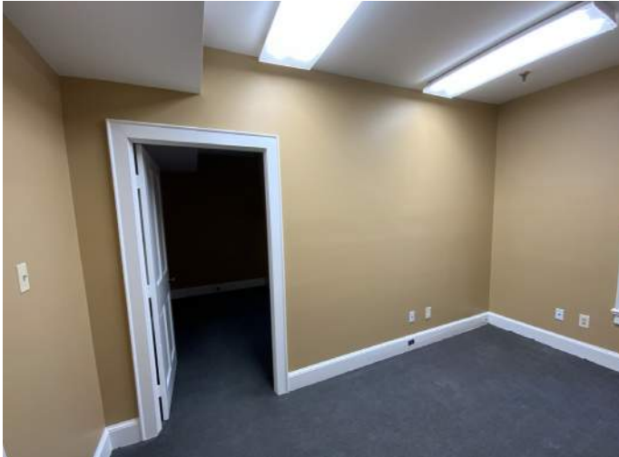
Office 314, South Elevation
