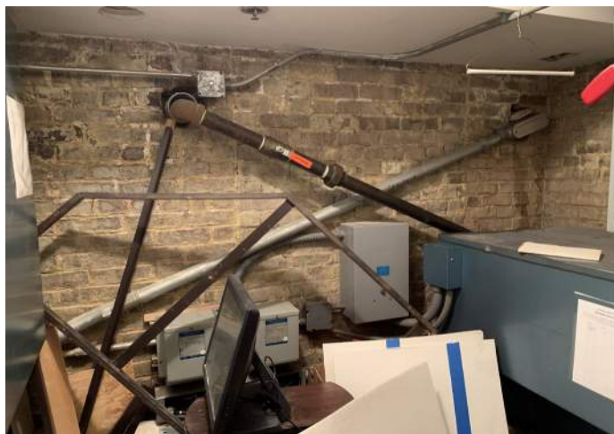
Elevator Machine Room 002B
