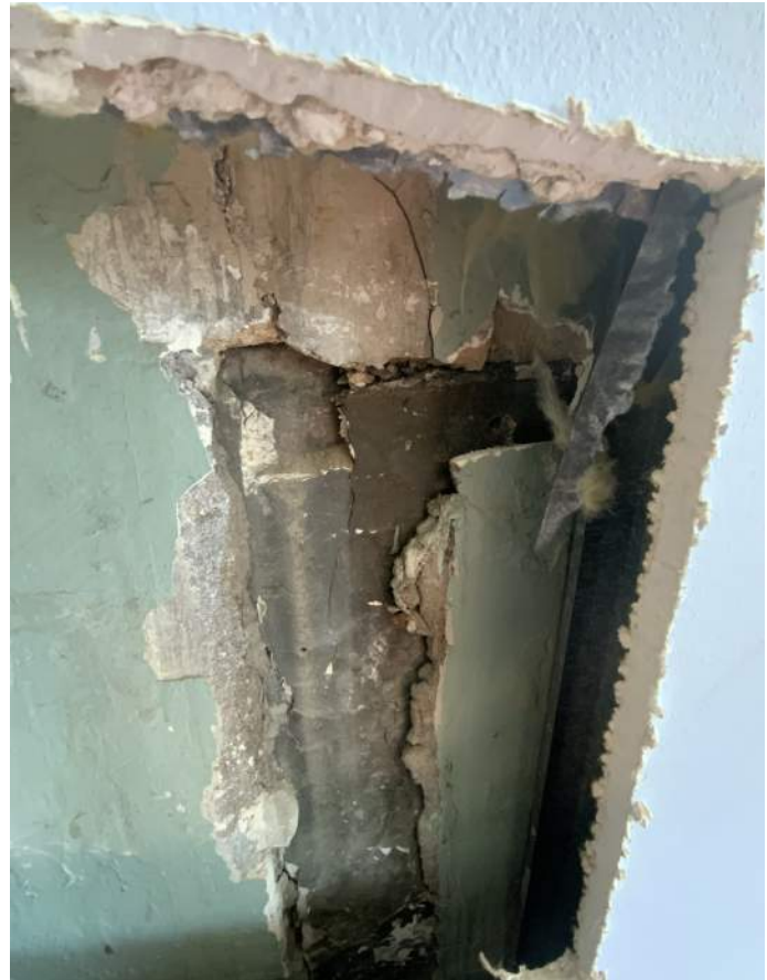
Figure PR5-2: Detail of historic plaster finishes found at investigative probe #5.
