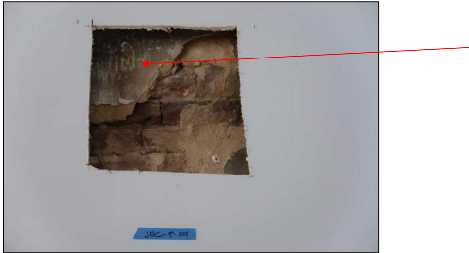
Figure 4: Probe #6 at west wall of second floor, Sample PT-201.
