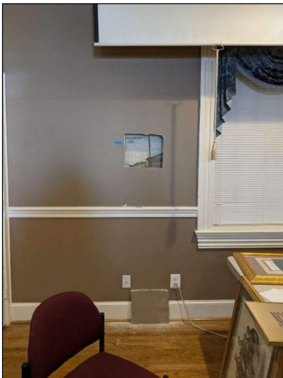
Figure 2: Probe #3 at north wall of the first floor, Sample PT-102.
