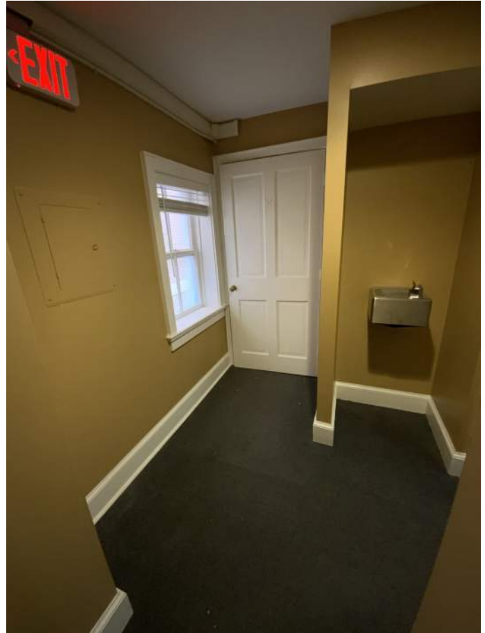
Corridor 205A, North and West Elevations
