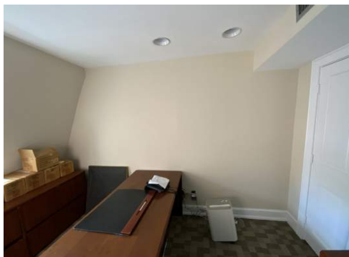
Office 404, East Elevation
