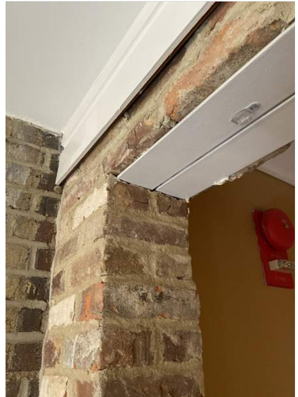
Figure 2D-9: Exposed lintel at corridor in front of elevator.
