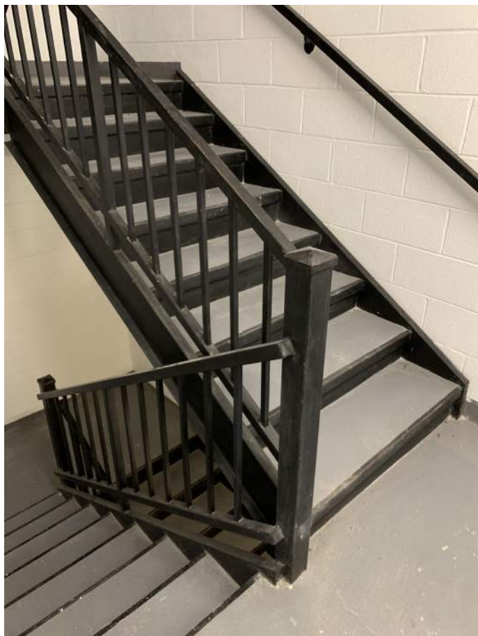
Stair 3, Typical Detail
