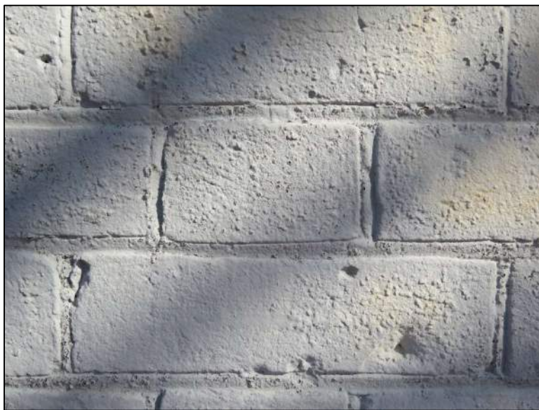
Figure 10: Detail of south facade pointing. Note the struck joint profile.
