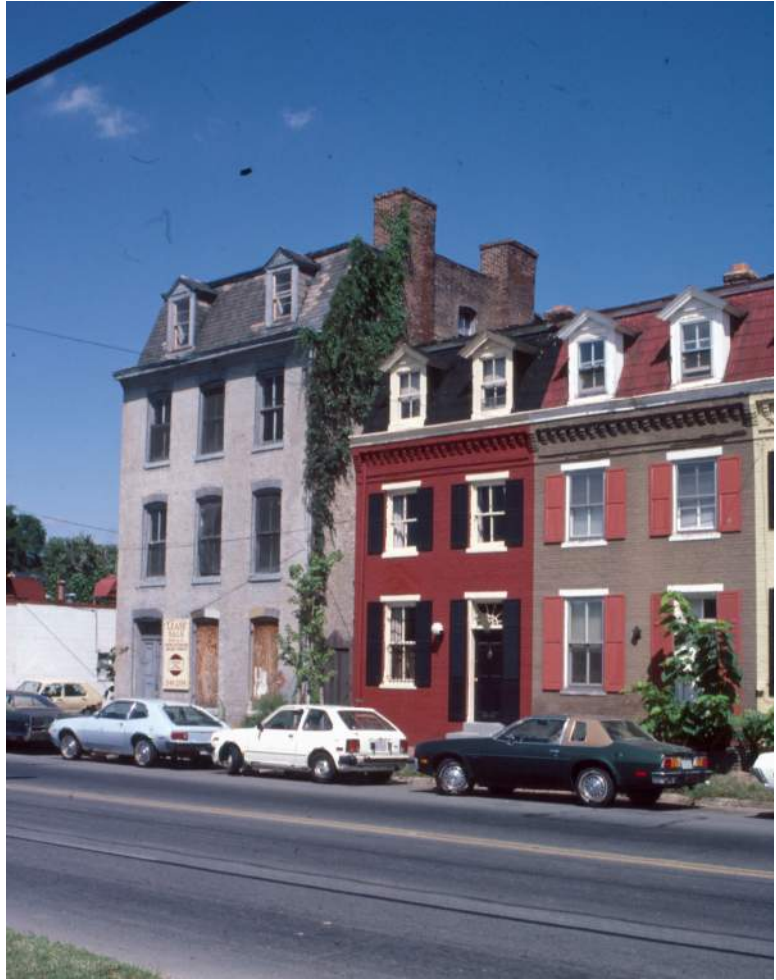
Figure 2B-19: View of 1315 Duke Street looking northwest from Duke Street, circa 1984. [Office of Historic Alexandria]
