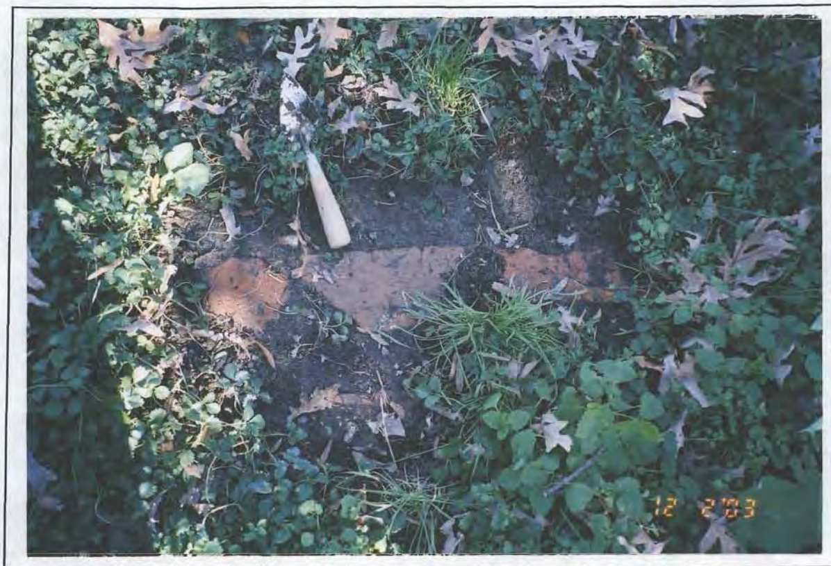
PLATE 13 Buried Foundation Wall visible in Exploratory "Cathole"
