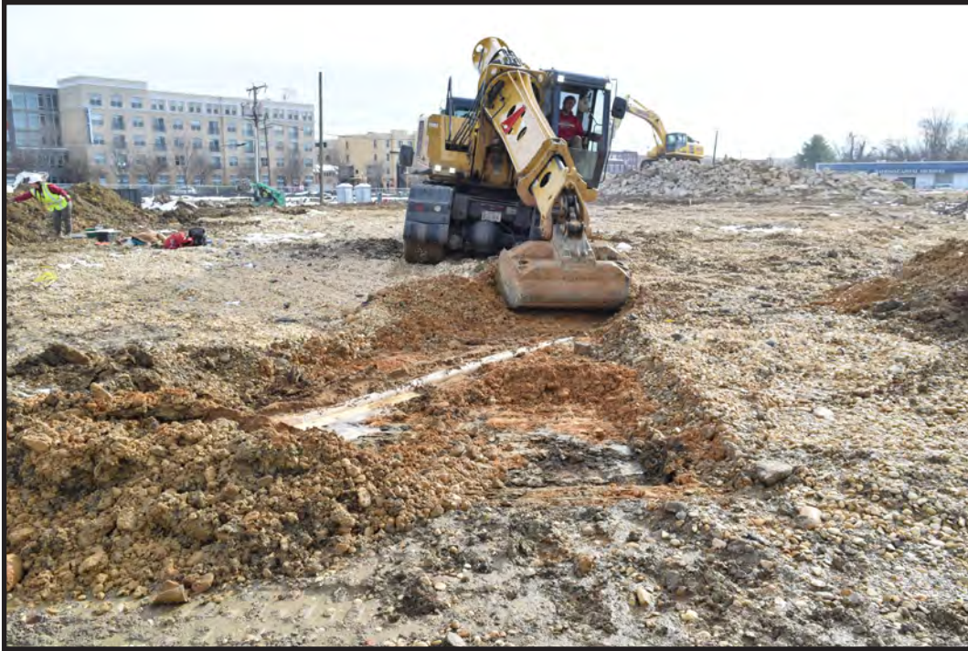
Figure 3.19 Photograph showing the start of excavation of Trench 2, view southeast (Goodwin & Associates staff, 1/6/2022). A plastic drainage pipe for the adjacent building's gutter is exposed in the northern end of the trench within the gravel layer for Building #2's concrete slab.
