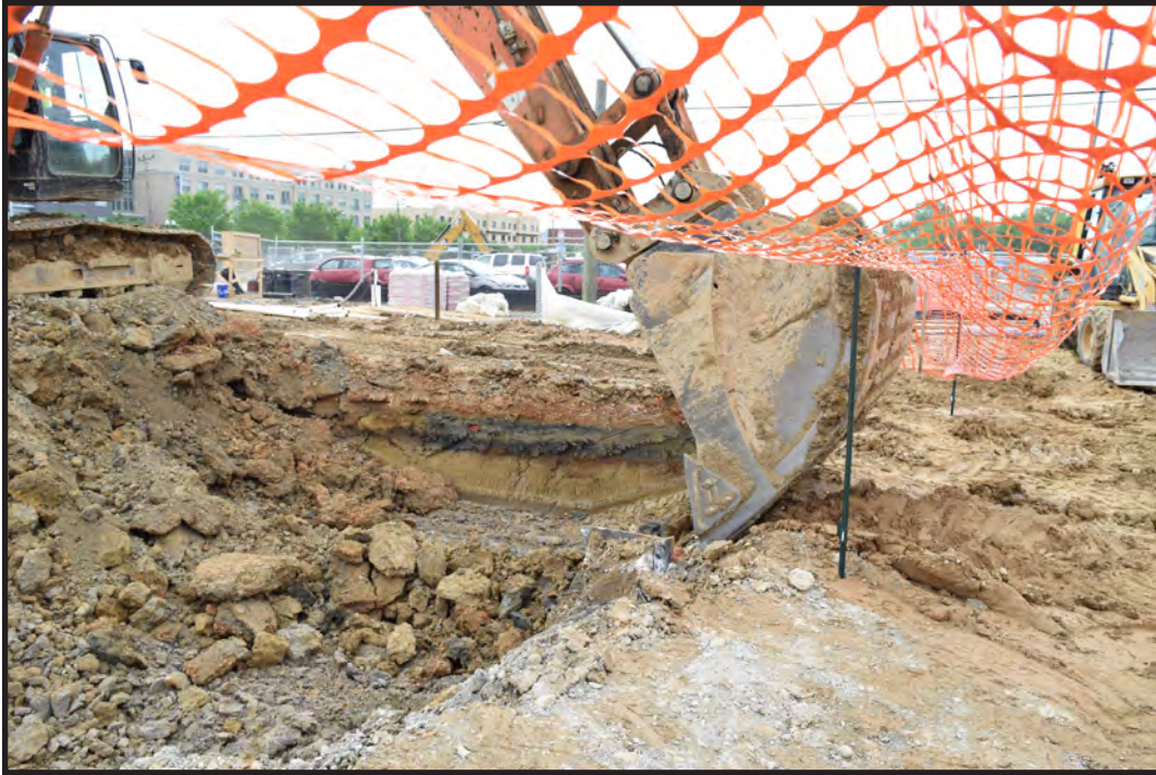
Figure 3.31 Photograph showing excavation of substrata following removal of VOC-impacted soil, view southeast (Goodwin & Associates staff, 5/17/2022). The VOC-impacted soil is visible in the profile as striated black and light yellowish brown silty clay deposits.
