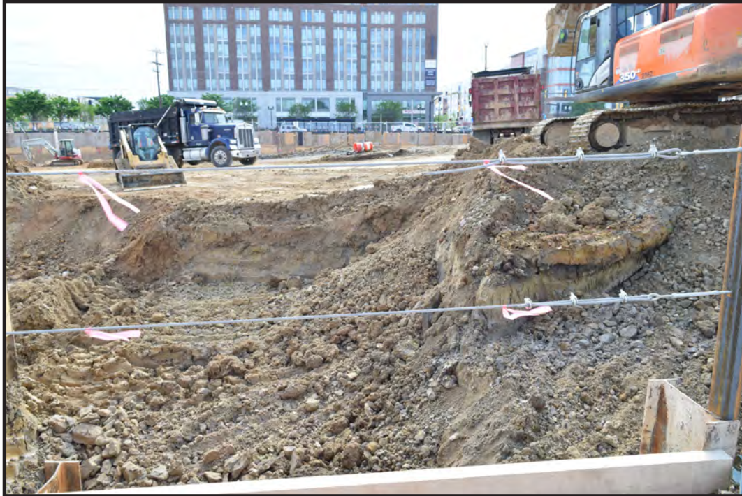
Figure 3.32 Photograph showing the VOC-impacted soil (foreground right) does not extend across the entire monitoring area (soil profile, background left), view northeast (Goodwin & Associates staff, 5/17/2022)
