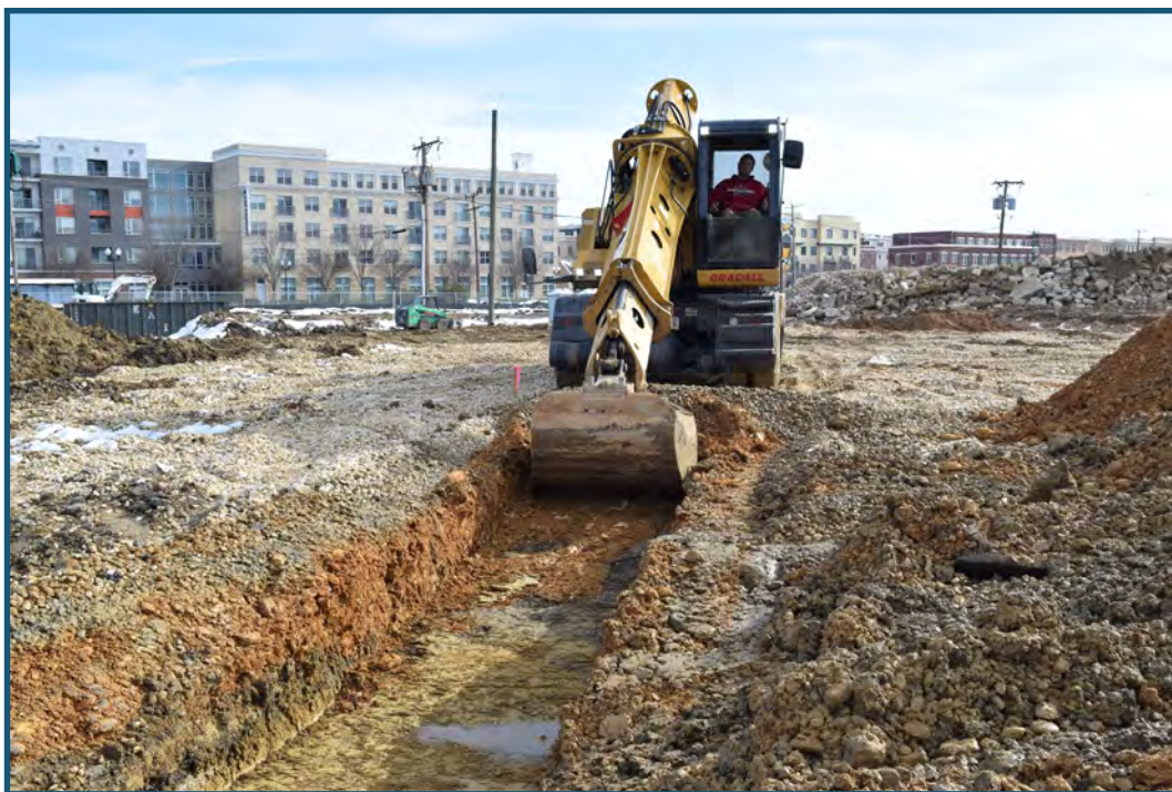
Figure 2.2 Photograph showing trench excavation using a Gradall, view southeast (Goodwin & Associates staff, 1/6/2022)
