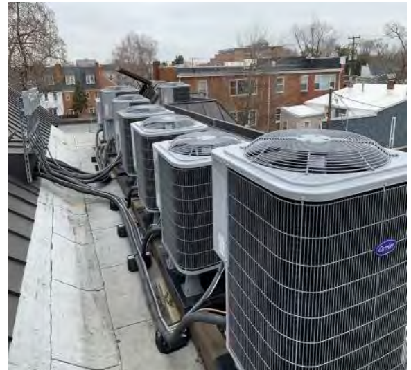
Figure 2D-17: Roof-mounted outdoor condensing units.
