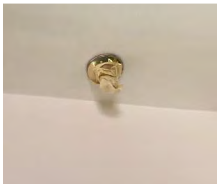
Figure 2D-33: Sprinkler head covered by masking tape.
