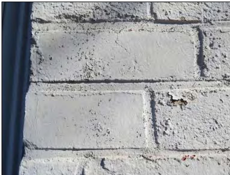
Figure 13: Detail of mortar at infill around windows. Note the smooth brick and the flat joint profile.
