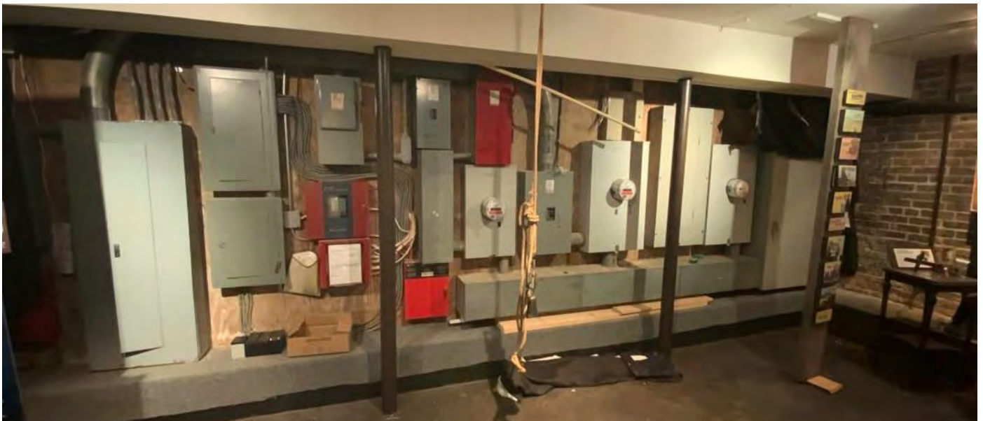
Figure 2D-27: Electrical Service Entrance Equipment – Basement Level
