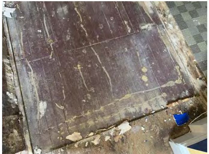
Figure PR16-2: Evidence of prior attic access through hinged panel in the floor.
