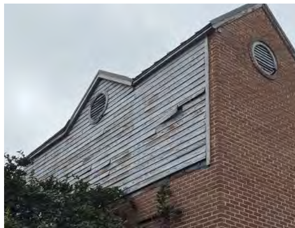
Figure 2E-7: Sheathing and siding damage at 1985 Addition (Period 5).
