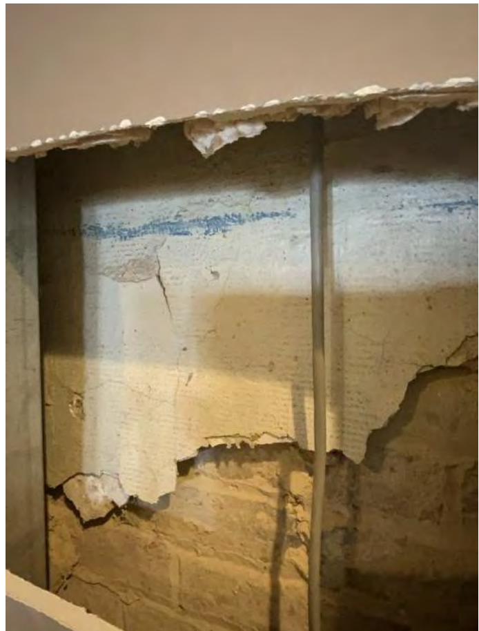
Figure PR3-2: Detail of historic 3-coat plaster found behind modern drywall finish.
