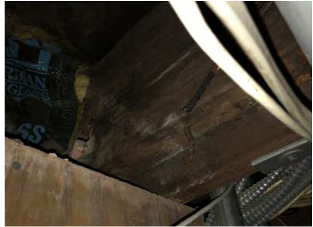
Figure 2C-4: Joist end visible from basement. Note the poor condition of the joists near the end.
