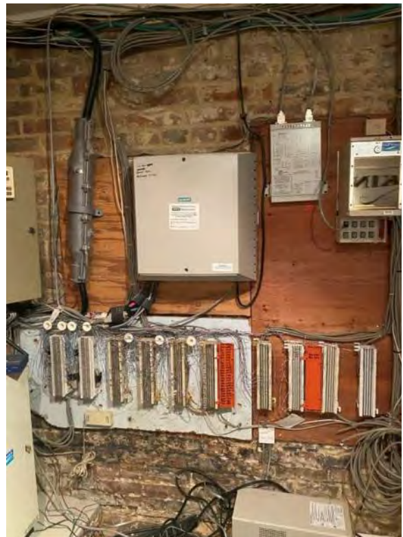
Figure 2D-29: Basement level patch panels.
