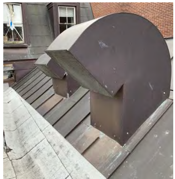
Figure 2D-20 Air intake and toilet exhaust
