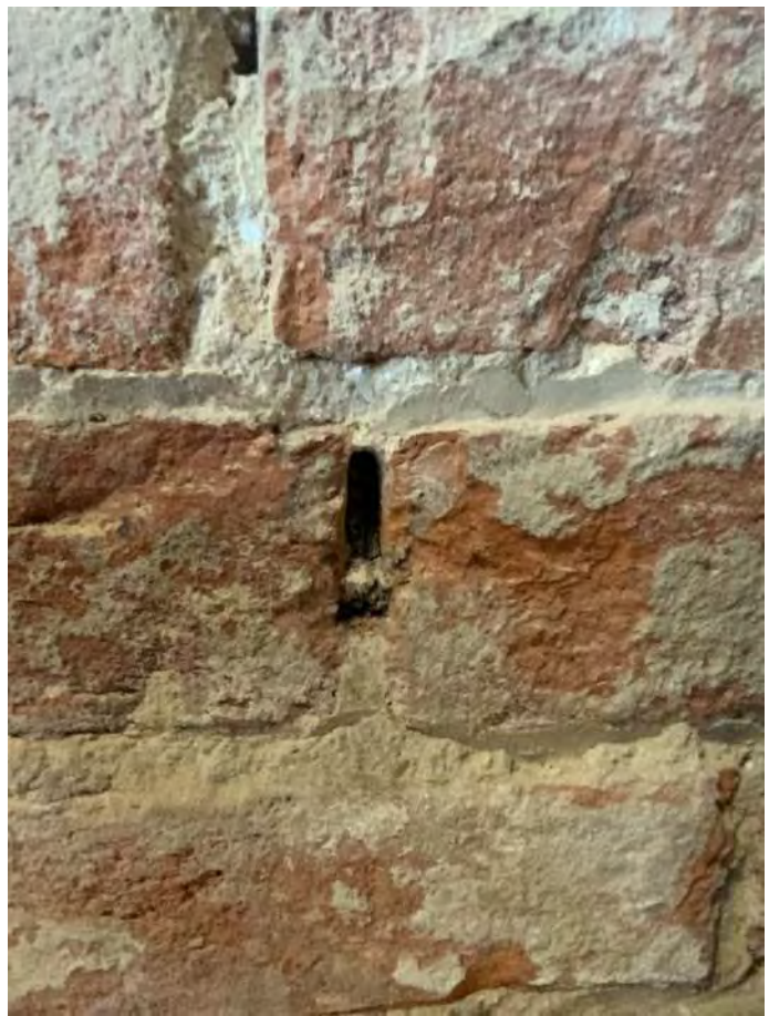
Figure PR1-4: Fragment of wood blocking found within the mortar joint.
