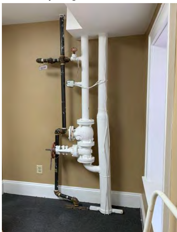
Figure 2D-32: 2-1/2" sprinkler riser with associated riser OS&Y gate valve and check valve located in the North Block.
