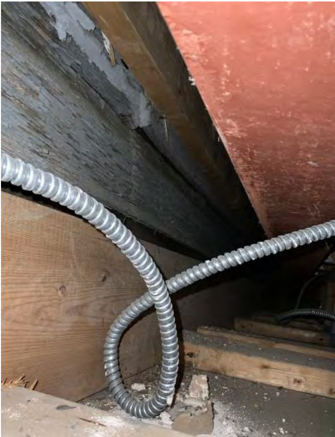
Figure PR9-1: View within probe #9 looking north locating the steel beam installed during the 1985 Addition and the remaining wood siding installed in 1937 per Permit #2415.
