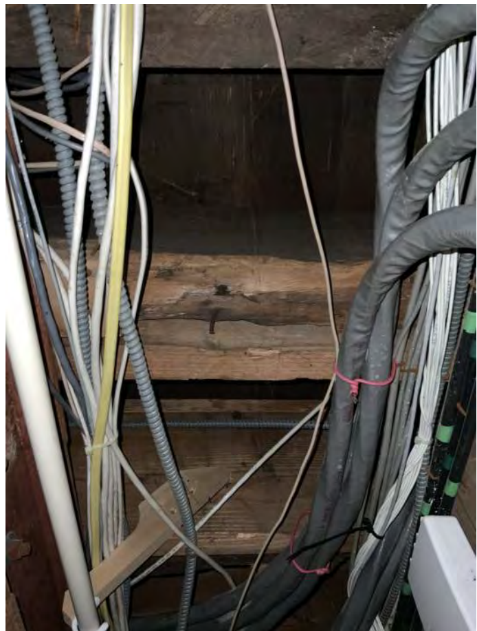
Figure PR19-2: Evidence of significant wood rot and deterioration at the bearing end of historic floor joists.
