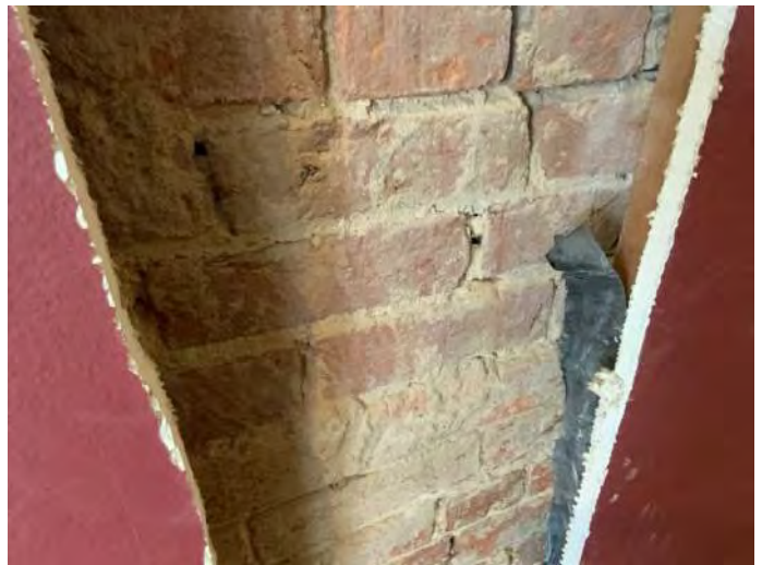
Figure PR1-2: One of two openings cut in existing drywall finish along west wall of Corridor 102. Existing wood stud framing found installed along historic brick masonry. A few cut nails were found within the mortar joints.
