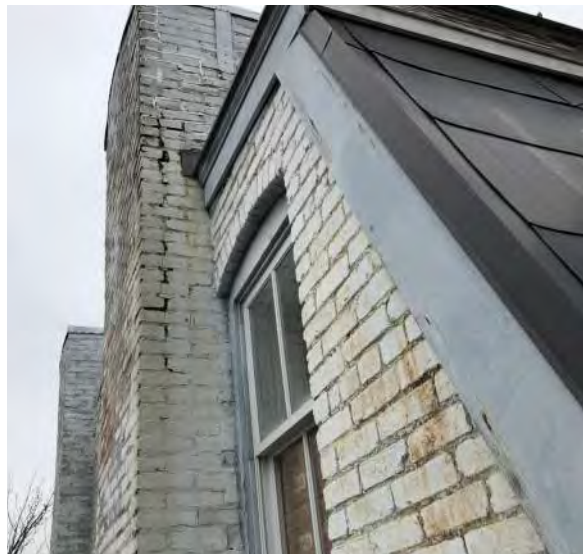
Figure 2D-14: Upper portion of east elevation of South Block; Note the poor condition of Chimney #2 and the prior repairs.
