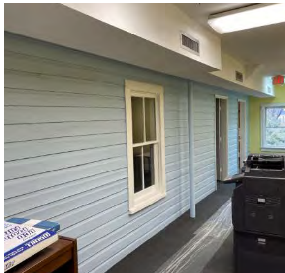
Figure 2D-30: Historic wood cladding on third floor wall at Central Passage and North Block.
