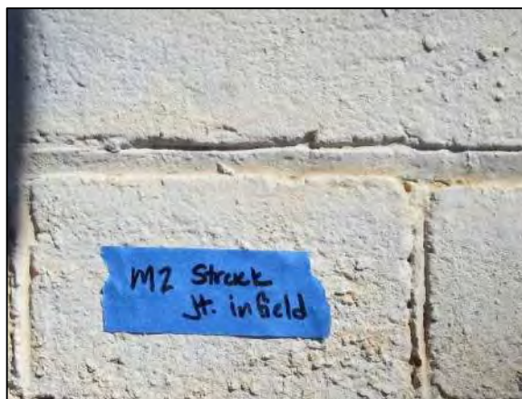
Figure 31: Location of Sample M-2. Note the crisp joint profile.
