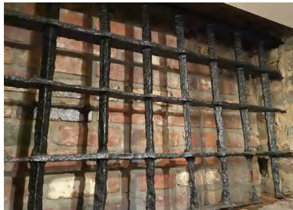
Figure 2C-14: Wrought iron grating within basement
