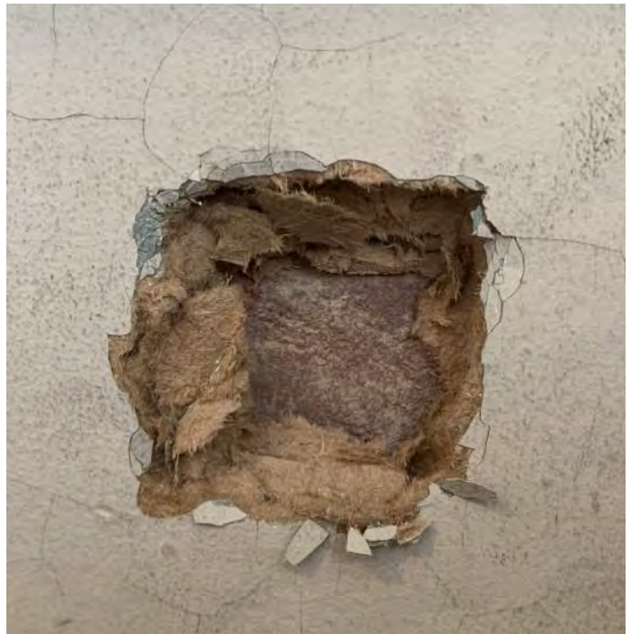
Figure PR2-2: Detail photo of wood fiber insulating board installed along historic brick masonry wall.
