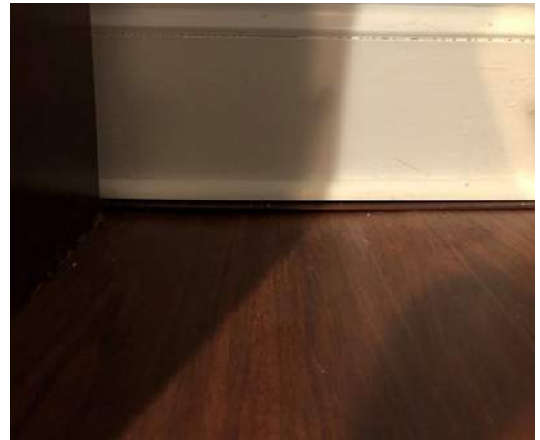
Figure 2D-5: Gap evident in baseboard trim at second floor office, opposite the corridor wall from Stair 1.
