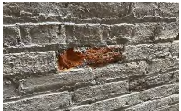
Figure 2E-3: Spall in brick masonry unit.
