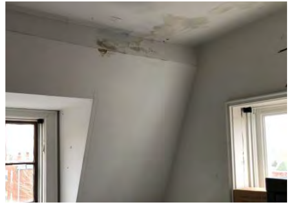
Figure 2D-8: Staining and bubbling of drywall finish in northeast corner of mansard roof within Office 403 in the South Block.
