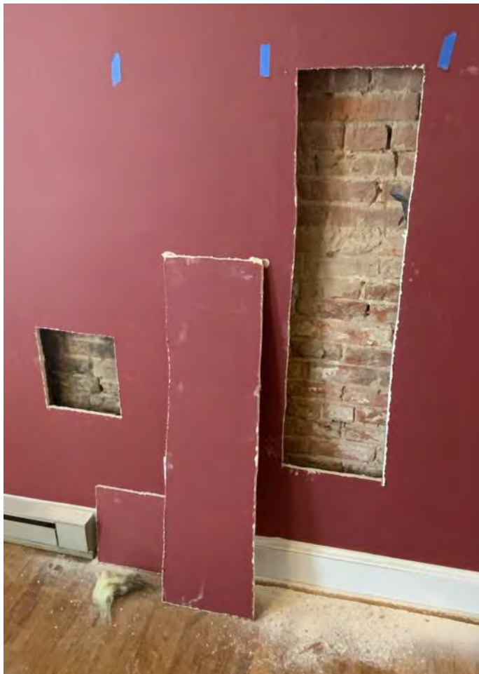
Figure PR1-1: Two (2) openings cut in existing drywall finish along west wall of Corridor 102.
