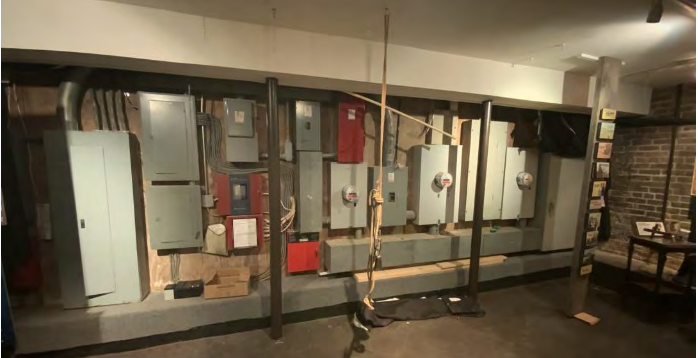
Figure 2E-9: Existing south wall of basement in South Block where the electrical service, panelboards, and other fire alarm and security devices are located.
