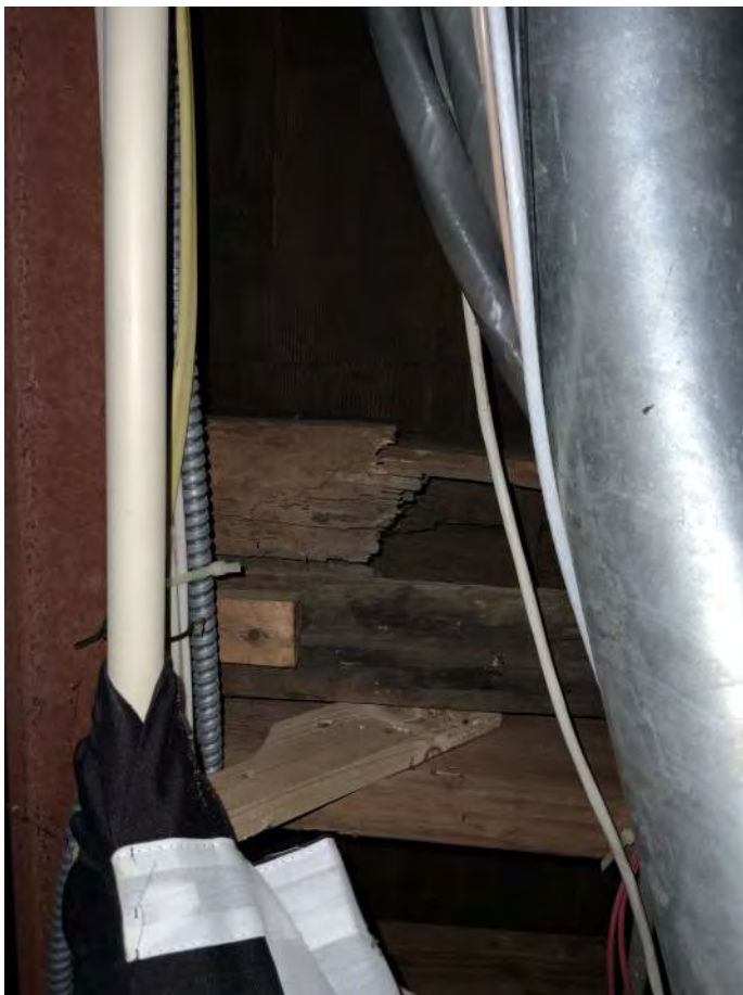
Figure PR19-1: Evidence of significant wood rot and deterioration at the bearing end of historic floor joists.
