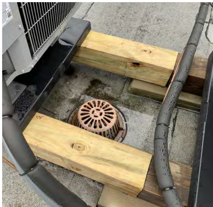
Figure 2D-25: Existing roof drain.
