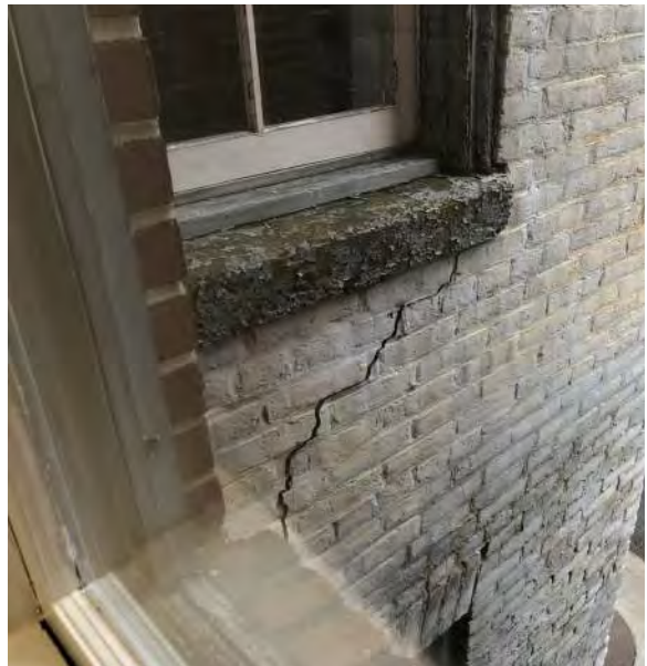
Figure 2D-12: Large crack at east return of North Elevation, located under masonry opening 219 of the North Block.
