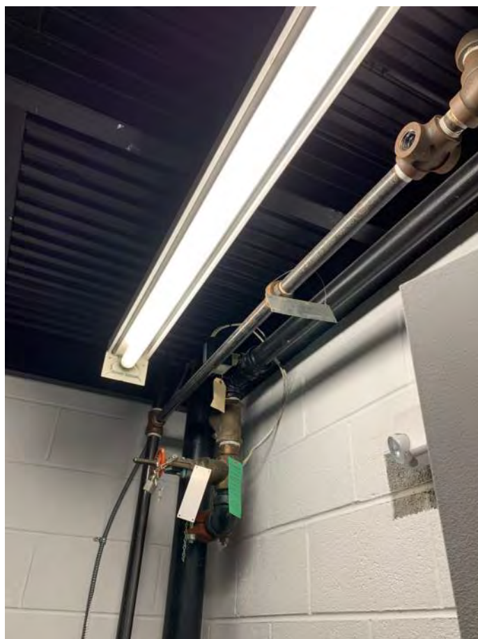
Stair 3, Standpipe in corner of egress stair
