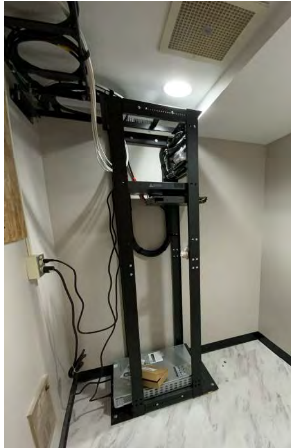
Figure 2D-28: Existing IT rack on second floor.
