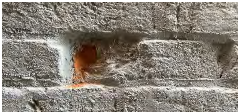
Figure 2D-13: Spalled brick face at west elevation.
