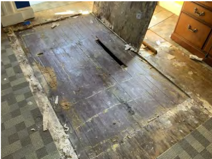
Figure PR16-1: Historic wood flooring uncovered from beneath a plywood subfloor and carpet tile.
