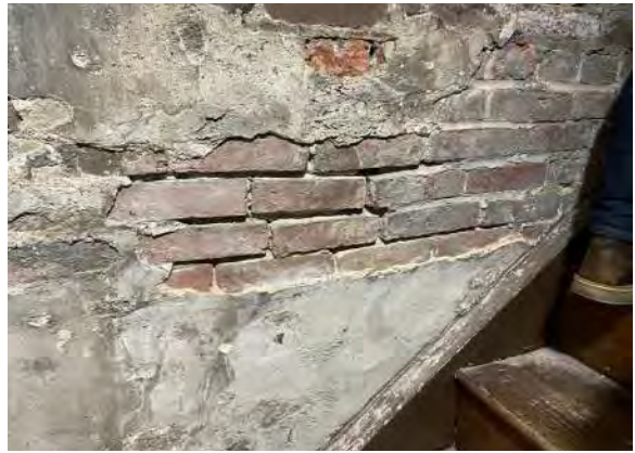
Figure 2D-11: Failing parge coat observed at east wall of Basement at Stair 1, located along west foundation wall.
