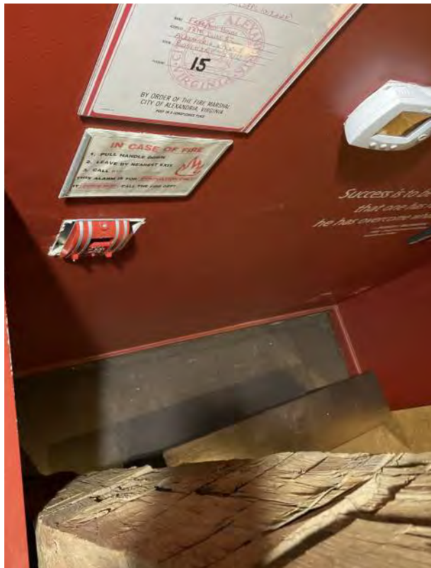
Figure 2D-38: Fire alarm manual pull station obstructed by exhibit at basement level.
