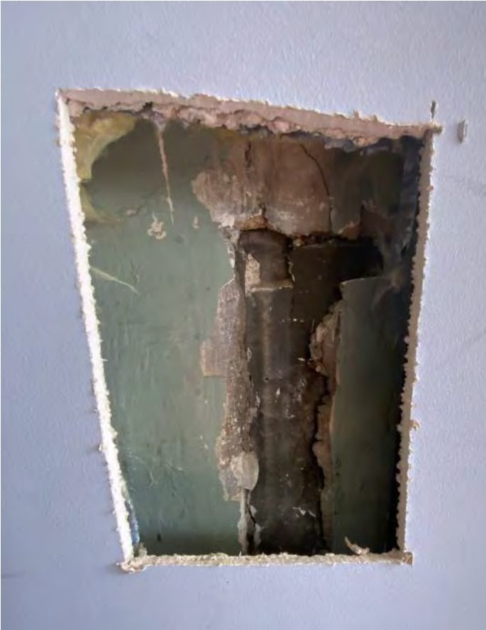
Figure PR5-1: Opening cut in existing drywall along east elevation of Conference Room 201 at the face of Chimney #1.
