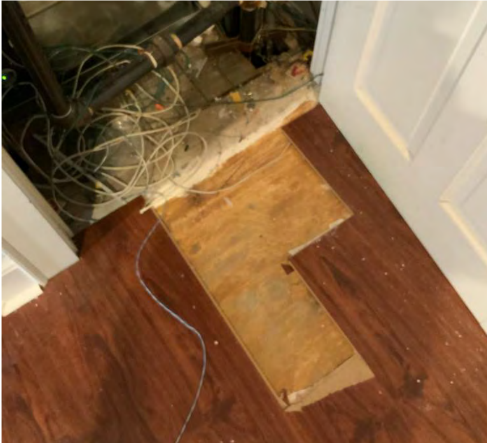
Figure PR8-1: Plywood subfloor uncovered beneath the existing laminate floor. The wood flooring in the adjacent mechanical closet may be original.
