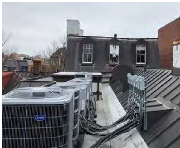
Figure 2C-10: Roofs viewed from the south end of the structure looking north. Note the flat roof of the 1980s addition, gable roof of the northwest portion, and mansard roof of the south portion.
