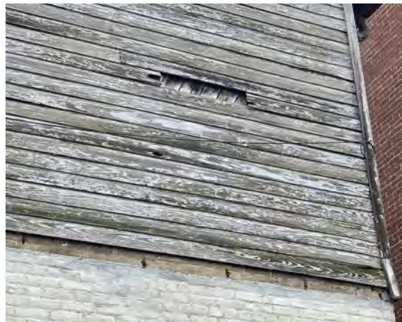
Figure 2E-6: Sheathing and siding damage at historic North Block (Period 4B).
