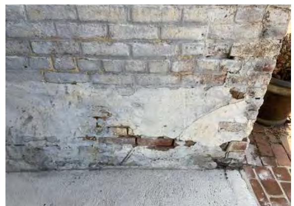
Figure 2D-10: Failed parge coat and mortar loss near grade at southwest corner of South Block
