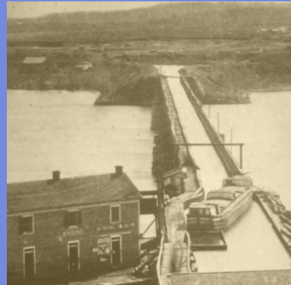
Aqueduct Bridge at Georgetown
