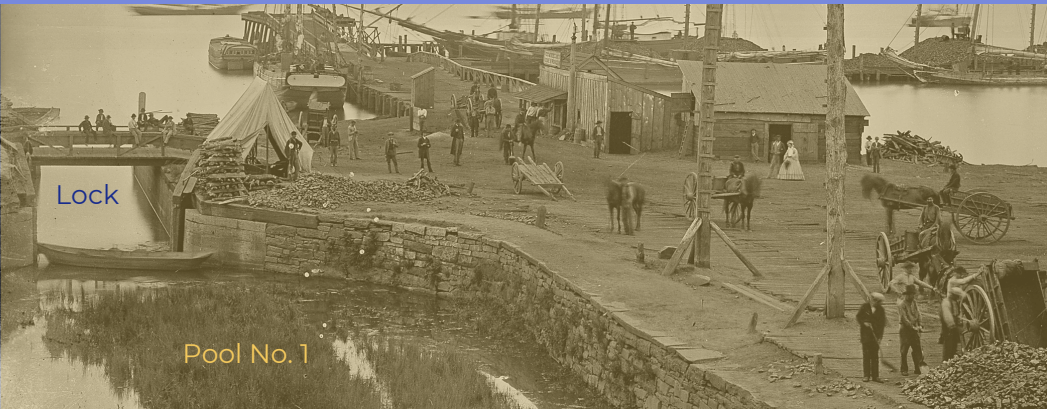
Alexandria Canal Lift Lock and Pool No. 1 on the Potomac River, ca. 1861-1865. Courtesy of National Archives.
