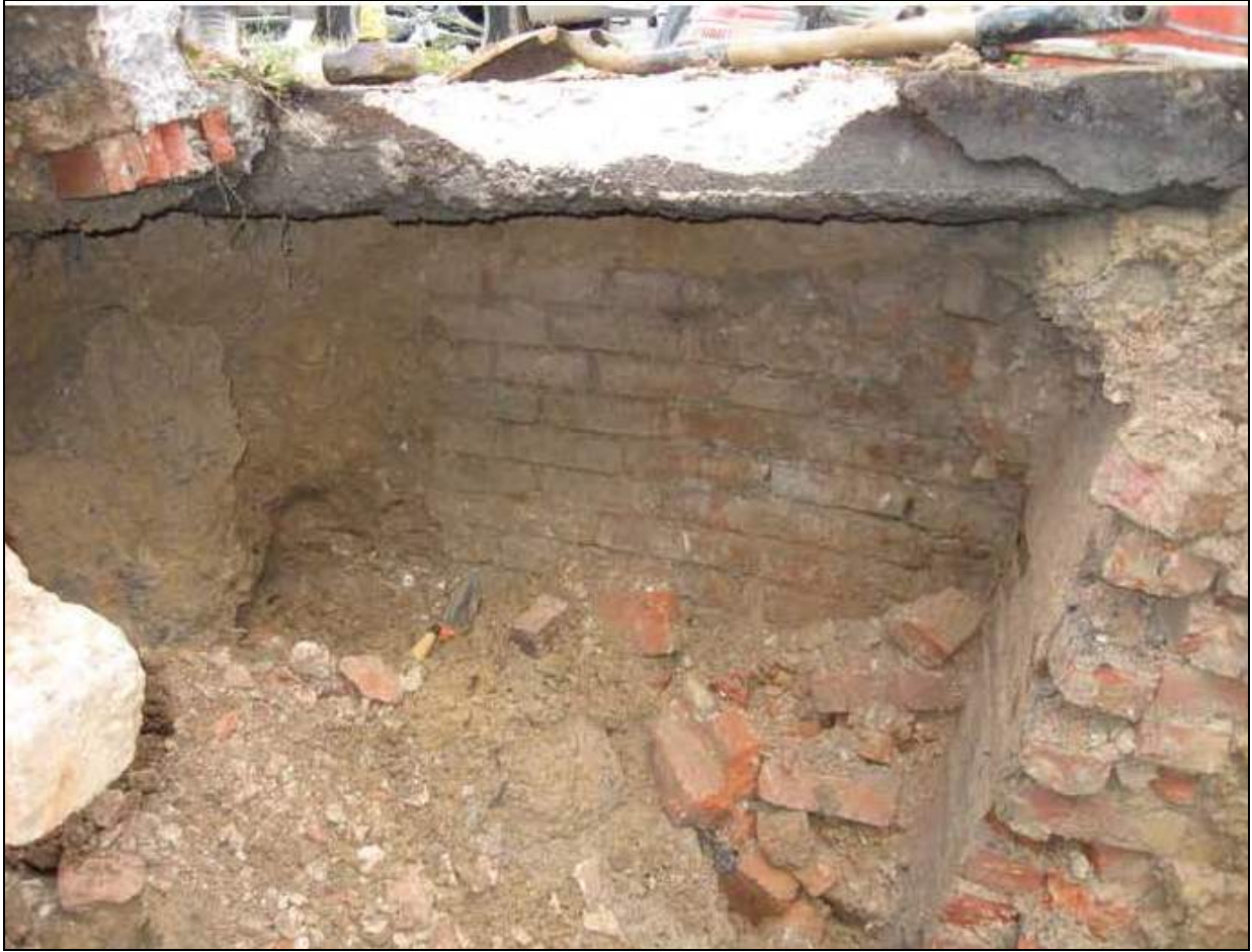
Northern Portion of Feature 3 beneath the Sidewalk, Pendleton Street.
