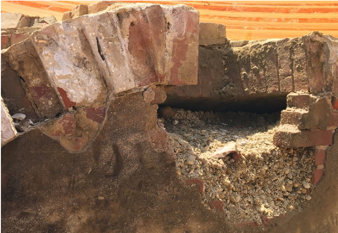
Figure 46: Close-up of Partition Wall showing Plaster
