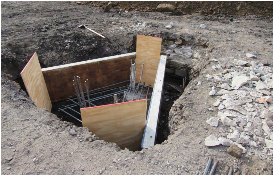
Figure 8: Concrete Form for Pile Cap
