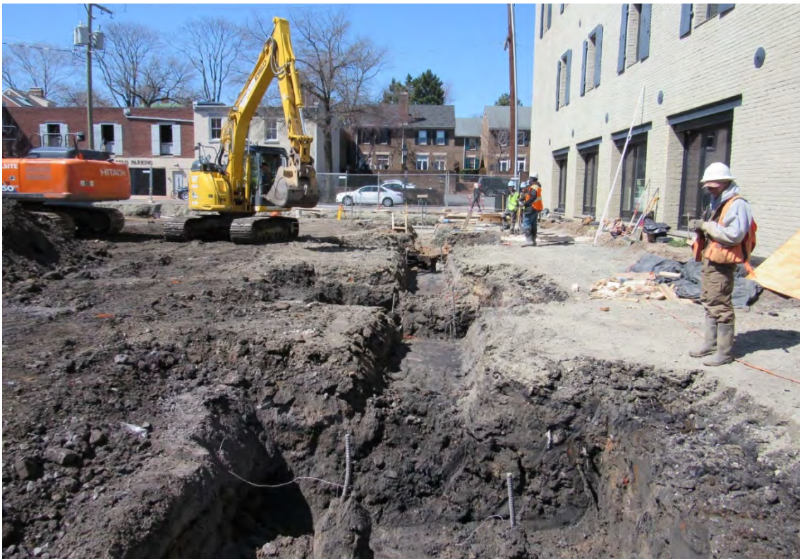
Figure 9: Example of Pile Cap and Grade Beam Trenching View West
