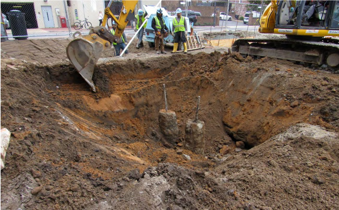
Figure 7: Excavation Around Augercast Piles Prior to Pile Cap Installation
