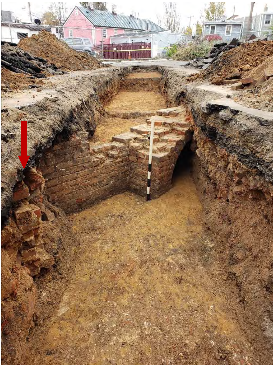
Photo 14: Detail of Relieving Arch and Portion of Interior Basement Wall (Feature 2), Facing Southeast. Red arrow marking section of interior wall.
