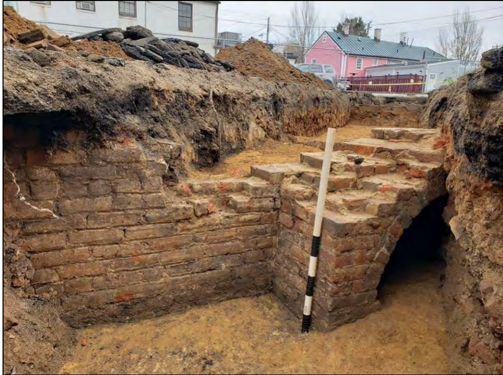
Photo 26: Overview of Exterior Wall and Relieving Arch, Facing Southeast.
