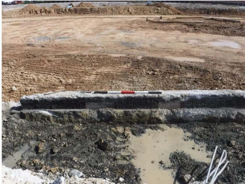
Figure 85: Feature 7 Interior Foundations Showing Possible Floor Joist Locations, View to East
