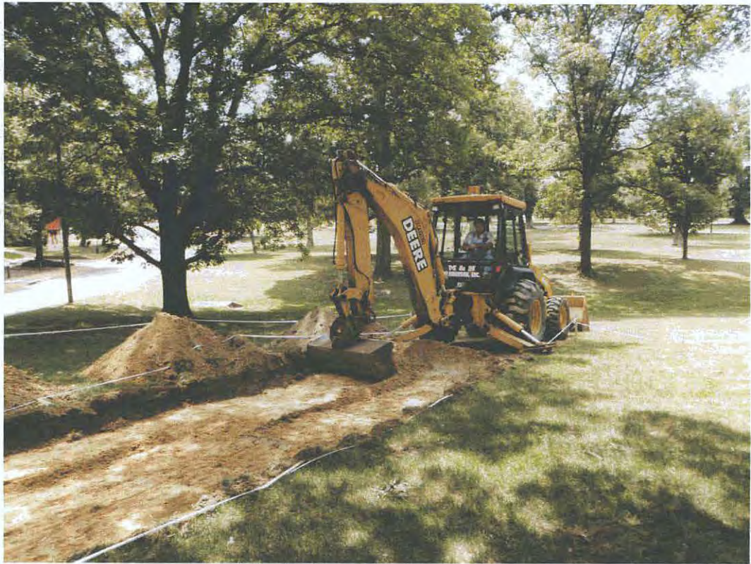
Figure 6. Mechanical stripping of Area 2 in progress, facing southeast.
