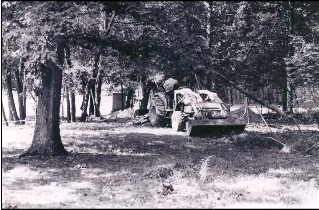
Figure 24. Mechanically stripping storm water detention area (Site 44AX173a).
