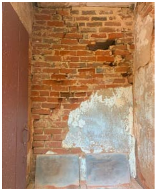
Figure 19j. Interior of West Privy (Room 116) looking east.
