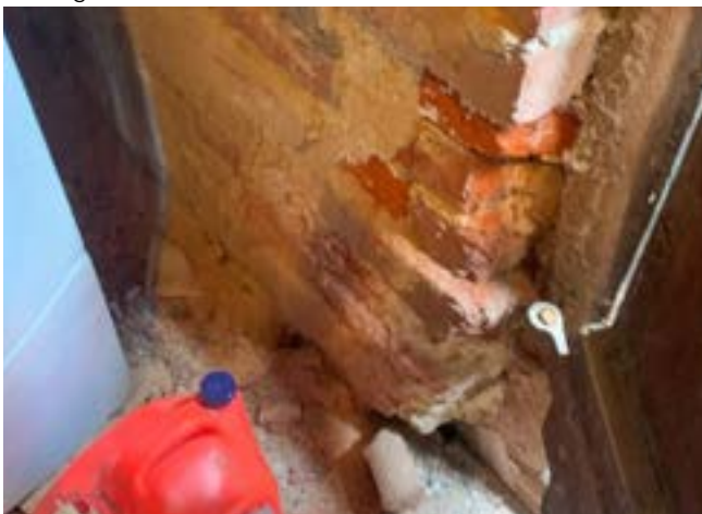
Figure 19g. Interior of the Smokehouse door looking northeast. (Room 115)
