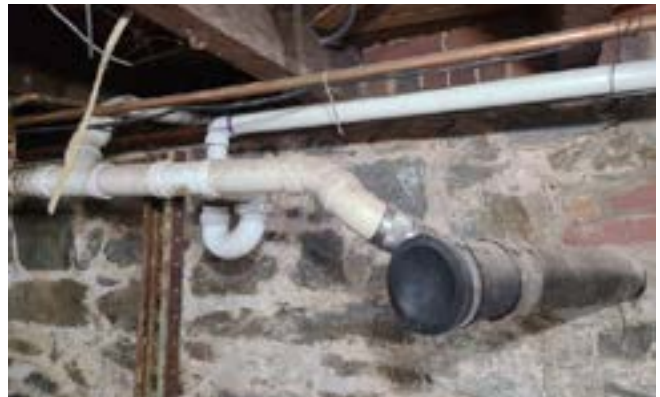
Figure 20aj. - Redirected Sanitary Line in Cellar
