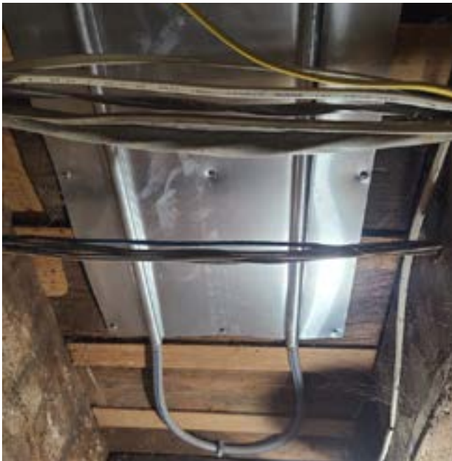
Figure 20k. - Underfloor Radiant Heating System
