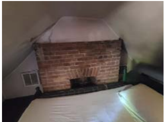
Figure 20f. - Supply and Return Air to Slaves Quarters
