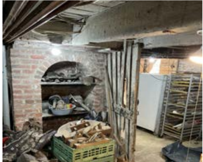
Figure 6a. - Added chimney base in the 1784 Cellar from the south.
