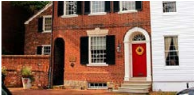
Figure 7s. - The original front grade may have been similar to that of Alexandria’s James Craik House of 1796 with its low cellar vents and plain steps protruding into the right of way.
