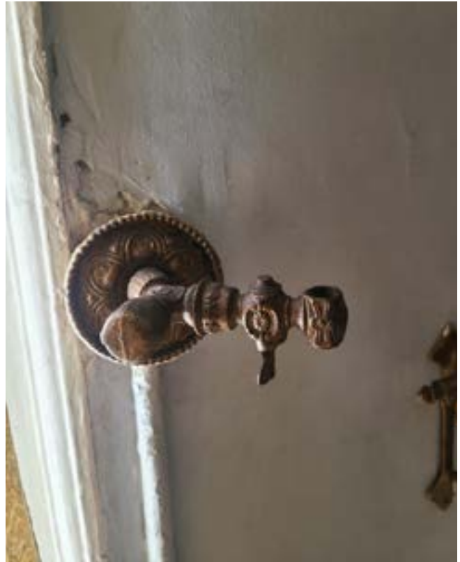
Figure 20r. - Remnants of A Second Gas Lighting Fixture
