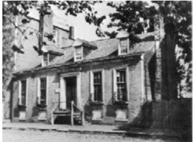
Figure 5e. - Lapped weatherboard seen at right end of a historic house in Alexandria ["The old Clapboard House on the John Dalton property and believed to the have been his house," Gay Montague Moore, Seaport in Virginia: George Washington's Alexandria , U Press of Virginia, 1949, 72].
