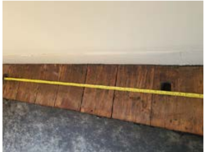
Figure 20b. - Previous Location of Cast Iron Radiators
