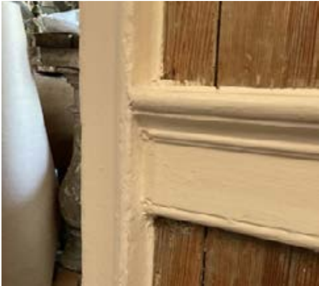
Figure 15n. - Chair Rail on the east side of the board partition between the Back Passage and Room 105 at the north jamb of the door.
