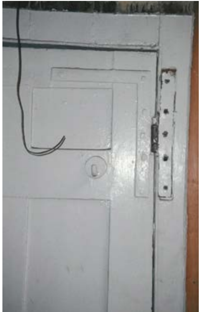
Figure 8j. - 2002 photo from the north of the door between the closet and the NE Chamber showing the back of the beaded vertical board partition and "HL" door hinge in place (Bierce Collection, Historic Alexandria).
