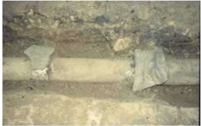
Figure 4c. - Drainage tiles, Photograph during archaeology in the cellar, 2000, Alexandria Archaeology [AX187_FR_68].
