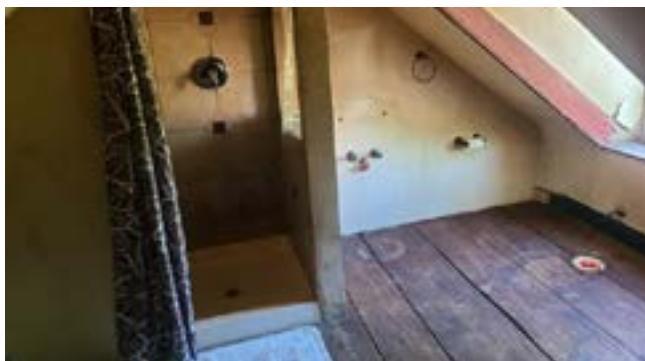
Figure 20al. - Shower and Demolished Plumbing Fixtures - Second Floor
