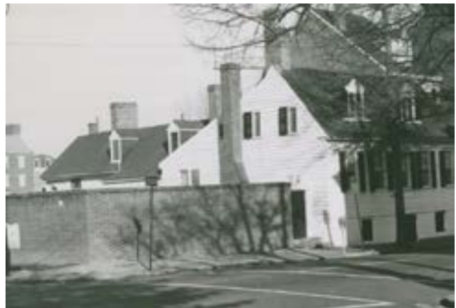
Figure 10f.- Murray-Dick-Fawcett House in 1975 showing the brick wall and garage before the construction of the courthouse (Special Collections, Alexandria Library). This photo also shows the chimney on the west wall from the 20th century boiler in the basement. The chimney was removed in 2002 by the former owner, who also lowered the brick garden wall by approximately 12".
