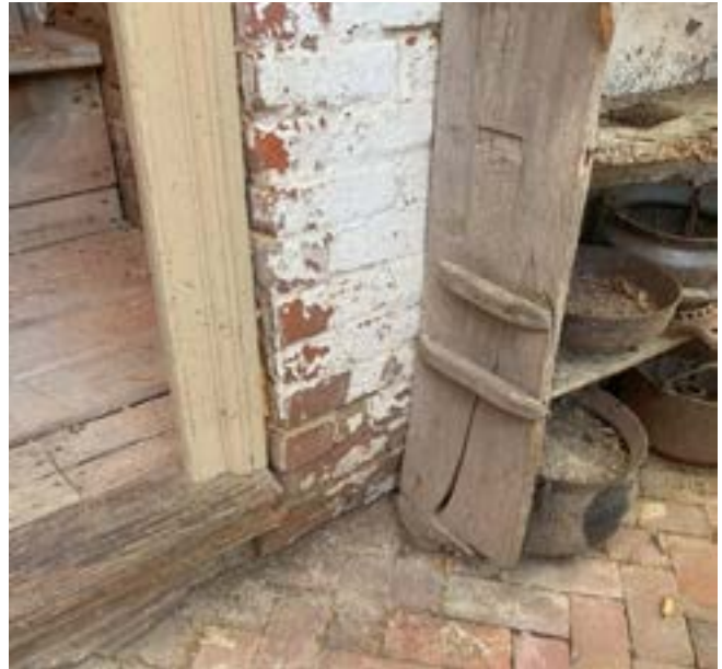
Figure 19l. West Privy, south jamb of door looking southeast.
