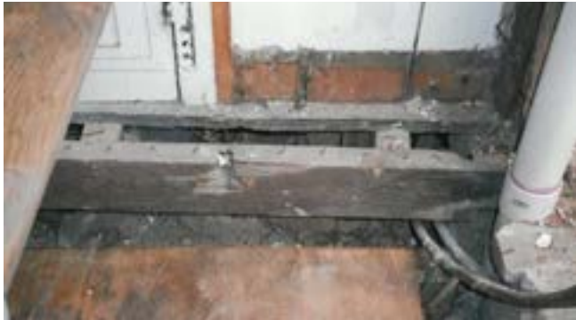
Figure 8l. - 2002 photo from the north of the vertical board wall between the closet and the NE Chamber. The floor joist is hewn (Bierce Collection, Historic Alexandria).
