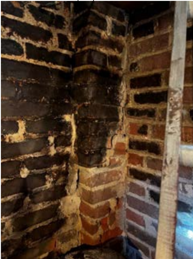
Figure 19i. Flue in the northwest corner of the Smokehouse (Room 115) looking northwest.
