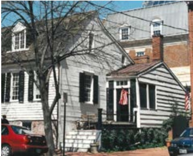
Figure 8g. - View from 2002 showing the continuous wide beaded siding on the east end of the east extension (Bierce Collection, Historic Alexandria).
