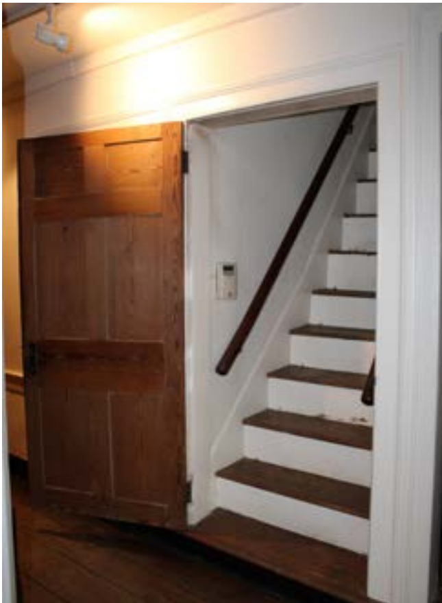
Figure 15j. - Stair 102 looking SE.
