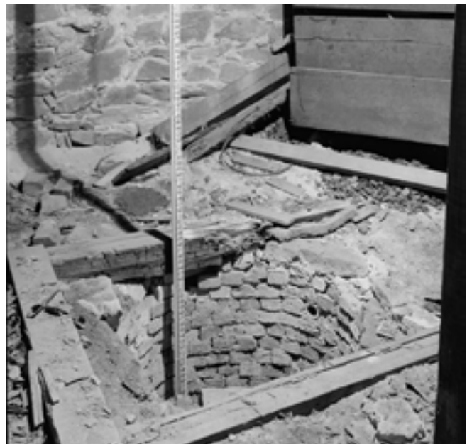
Figure 7q. - Cellar, view of the cistern with scale, HABS, 1936. The wood frame probably previously held a cover over the opening.
