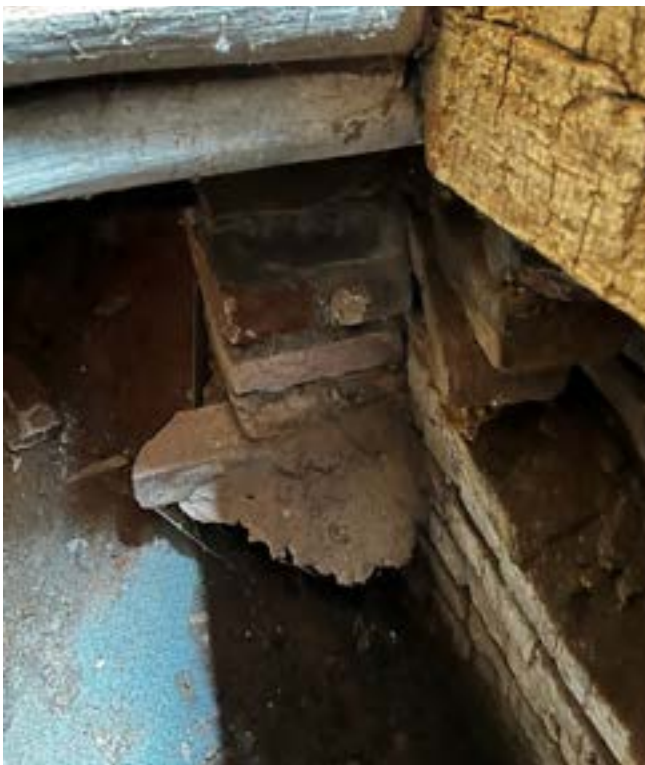
Figure 19m. North Privy with floor removed looking to northwest.
