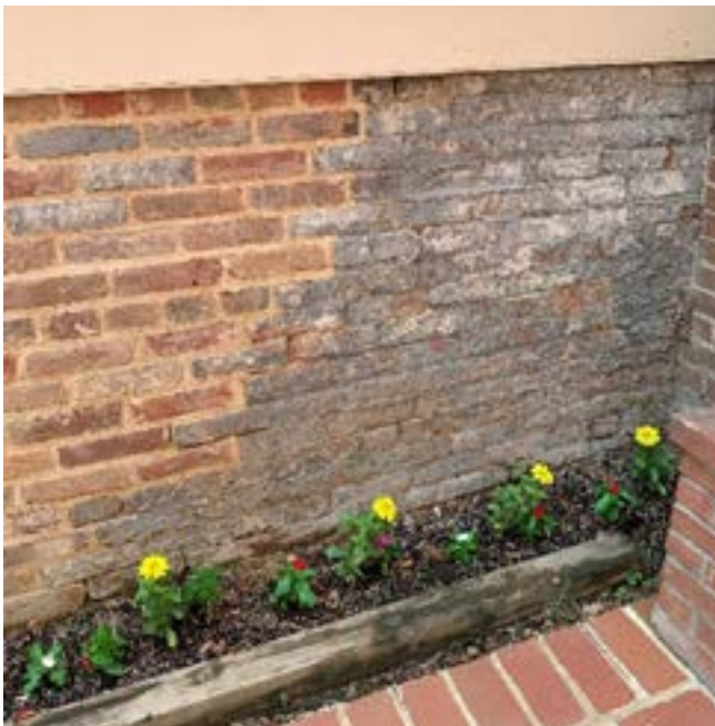
Figure 19o. East side of the 1816 extension looking east.
