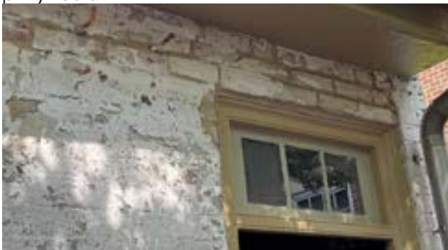
Figure 19k. Head of door to East Privy (Room 118) looking northwest.
