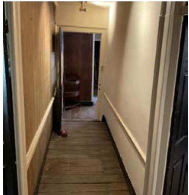
Figure 15o. - Back Passage looking north.
