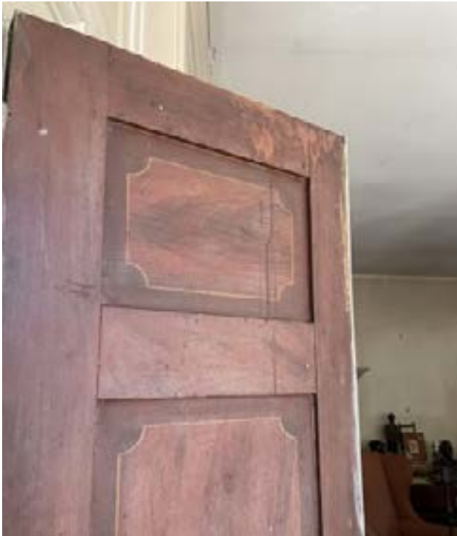
Figure 15i. - Decorative graining on the interior of the southern cupboard door in the Hall.
