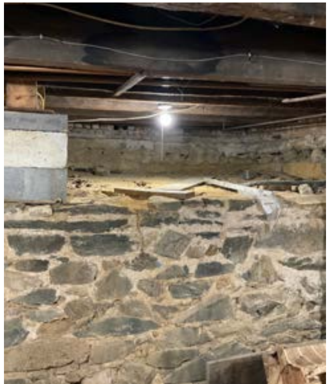
Figure 15l. - Crawl space looking SE under 1784 section.
