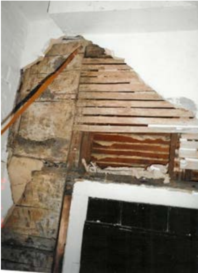
Figure 9f. - 2002 Photo from N of the former window in the N wall of the NW Room from the enclosed porch showing the inserted door and scored flush board and plaster (Bierce Collection, Historic Alexandria).
