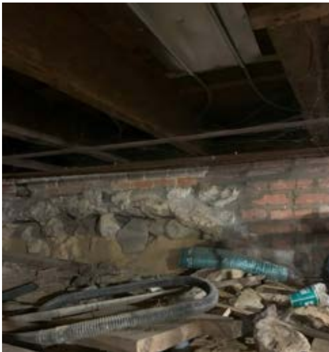
Figure 19c. Foundation below the east end of the 1874 section looking south (Room 003)
