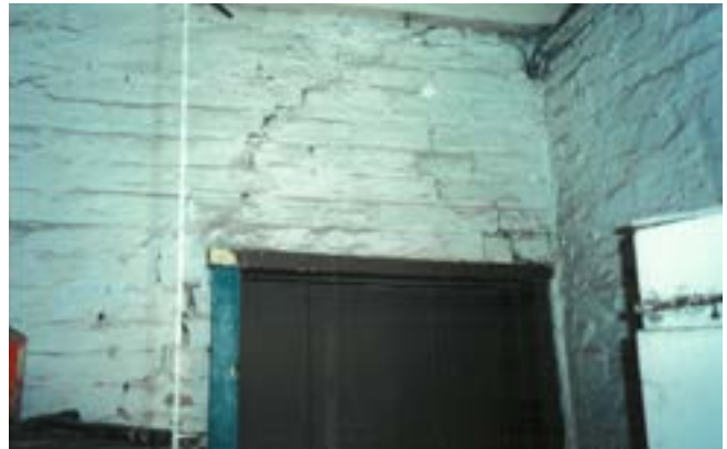
Figure 7f. - Head of Door connecting room 114 and room 113.
