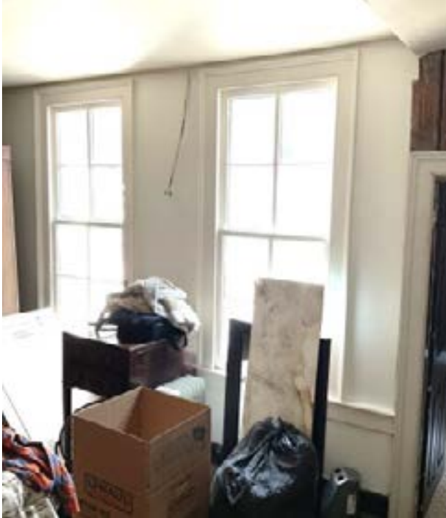
Figure 15q. - North wall of Room 107 looking northwest showing rebuilt windows and ceiling.
