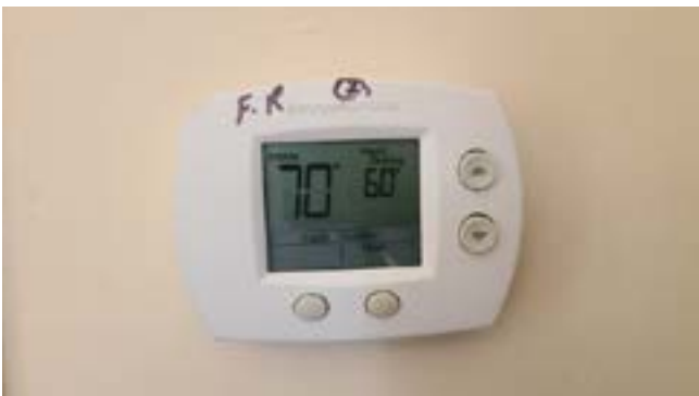
Figure 20o. - Typical Hydronic Zone Room Thermostat
