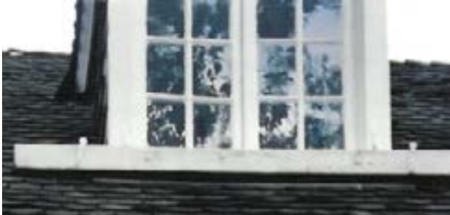
Figure 15b. - Detail, South Elevation, eastern dormer with shutter attachment bar at bottom, Bierce Collection, c2001.
