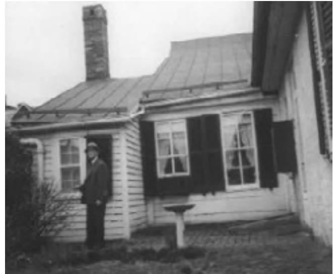
Figure 10h. - C. 1960 photo of Lewis Hooff at the rear of the house showing the closet of the 1816 extension and the two mid-19th-century windows, Historic Alexandria, Alexandria VA.
