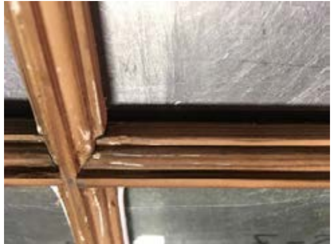
Figure 15a. - Interior detail of muntin. Typical south window sash during restoration.
