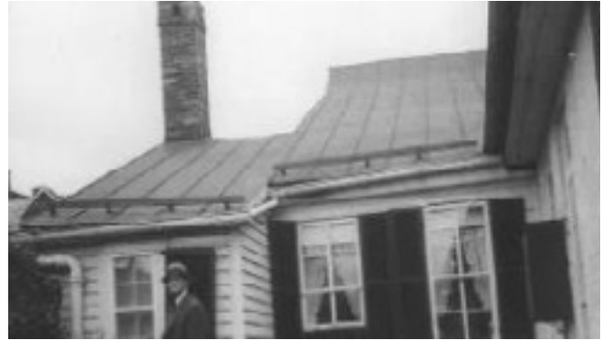
Figure 9g. - Snow brake irons supporting wooden board shown on the north slopes of the 1784 and 1816 sections in c1960, Historic Alexandria, Alexandria VA.
