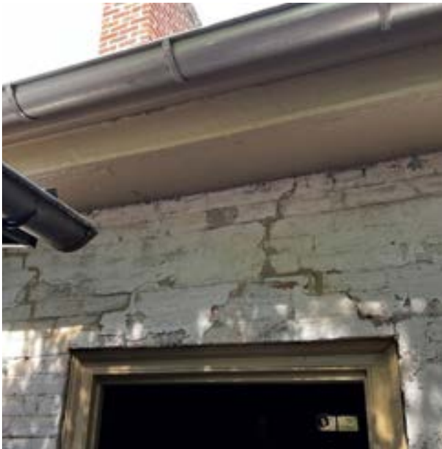
Figure 19f. Doorhead at the Smokehouse (Room 15) door looking west.
