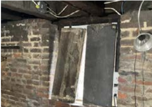
Figure 15g. - Interior of south wall at east bay.
