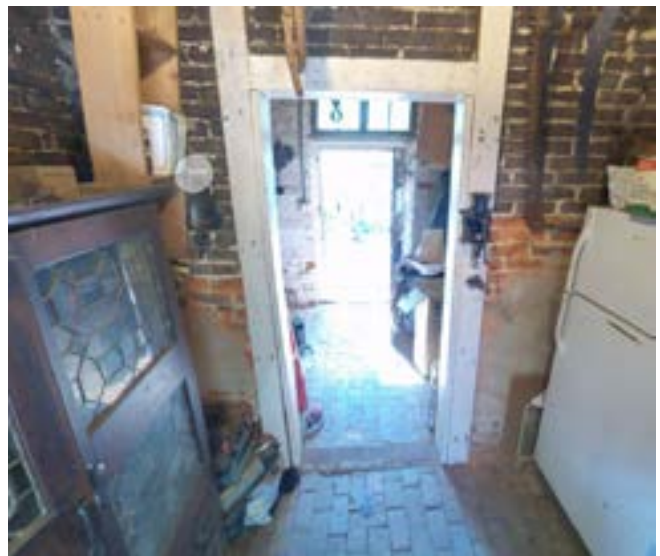
Figure 19h. Door between the Smokehouse (Room 114) and the Service Room (Room 115).
