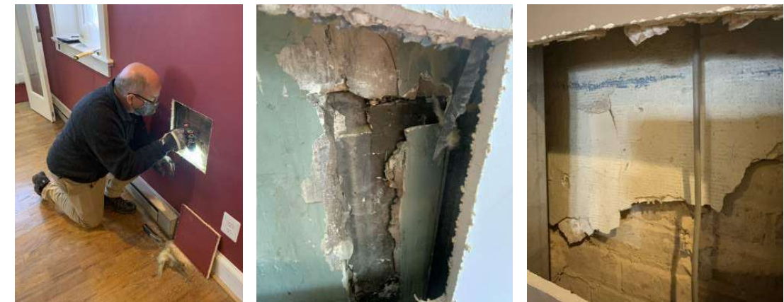
Figure 02: Images showing process of investigating behind existing modern drywall finishes to uncover evidence of historic 3-coat plaster.
