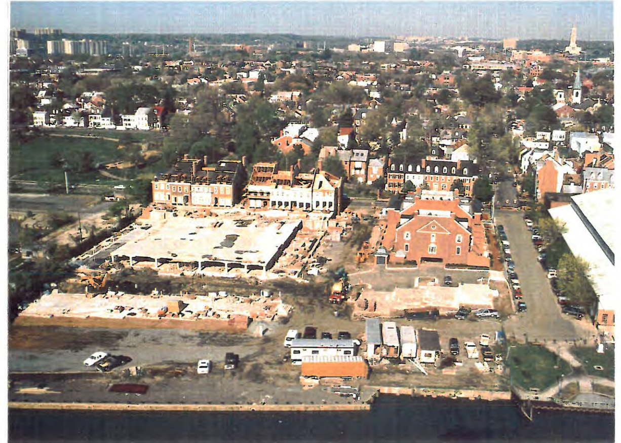
Harborside townhomes under construction in the spring of 1991.
