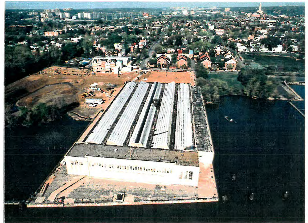
Construction at Old Ford Plant site in the spring of 1991.
